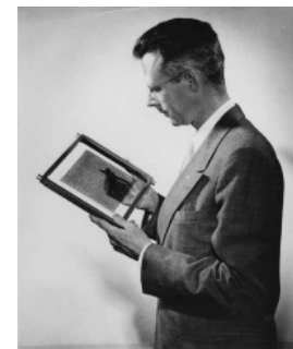
B.2.8. Jay Forrester holding a frame of core memory from the Whirlwind computer. He invented magnetic core memory while working at MIT in the early 1950s. His invention proved much faster and more reliable than the earlier Williams Tubes or delay-line memory technologies.
