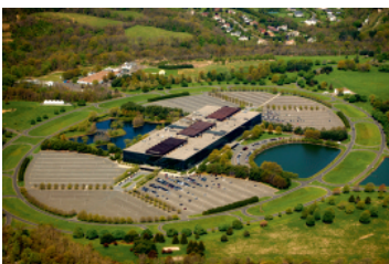
Fig. 7.1. An aerial view of AT&T Bell Labs in Holmdel, New Jersey. The building was designed by the architect Eero Saarinen and for forty-four years it was the home of an advanced research laboratory owned successively by Bell Telephone, AT&T, Lucent, and Alcatel.
