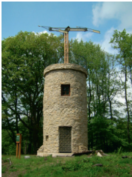
Fig. 10.3. One of Claude Chappe's telegraph towers was rebuilt near Saarbrücken, in Germany. The French engineer Chappe succeeded in covering France with a network of 556 stations stretching a total distance of 4,800 kilometers. The network was used for military and national communications from 1792 to the 1850s.
