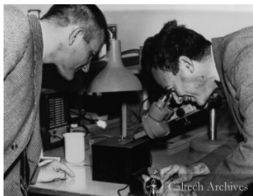
Fig. 15.1. Richard Feynman examining Bill McLellan's miniature electric motor in 1960. The motor could generate a millionth of a horsepower and Feynman paid McLellan the $1,000 prize money.
