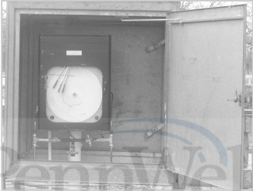
Fig. 9–9. Gas well meter. The volume of gas sold is calculated from pressure recorded on paper charts like that shown here. The charts are collected regularly by the lease operator and read by technicians at the company office.
