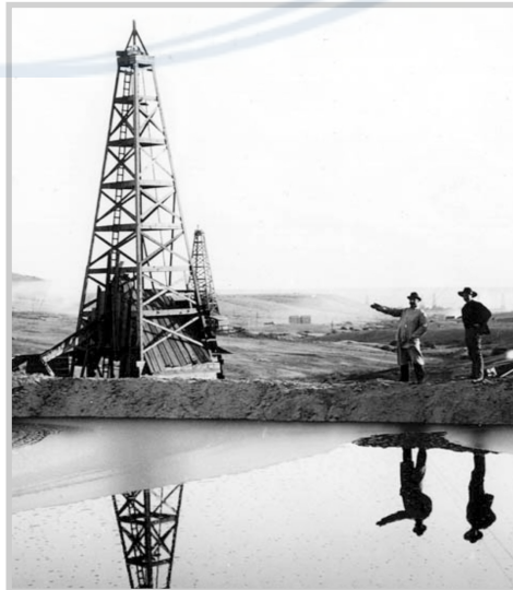
Fig. 1–1. Oil sump at Spindletop, ca. 1902. Oil sumps were open to the air, and much of the gasoline and naphtha just evaporated. Producers didn't mind—the internal combustion engine had not been invented yet. They were after the kerosene. Courtesy of Spindletop Museum.
