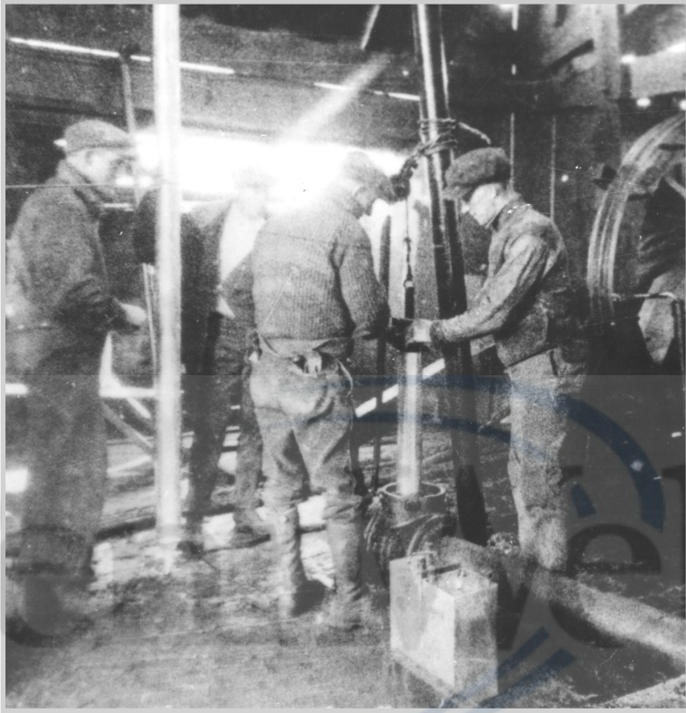
Fig. 1-4. Drillers lowering a torpedo into a well in 1922. Drillers to the left hold another torpedo. The pipe to the right handles the flow immediately into a tank. Courtesy of Southwest Collection, Texas Tech University.
