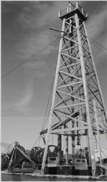
Fig. 5-2. Cable tool rig from the 1920s. Courtesy of Canadian Petroleum Interpretive Centre.
