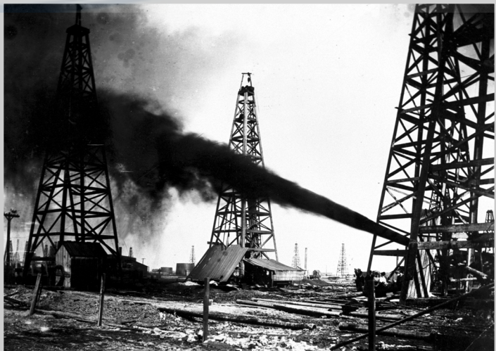
Fig. 6–1. Controlled blowout at Sour Lake, Texas. Courtesy of Spindletop Museum.
