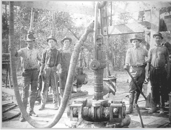
Fig. 1-7. The first rotary drilling job. Rotary drilling came to the U.S. first at Spindletop in 1901. Courtesy of Spindletop Museum.
