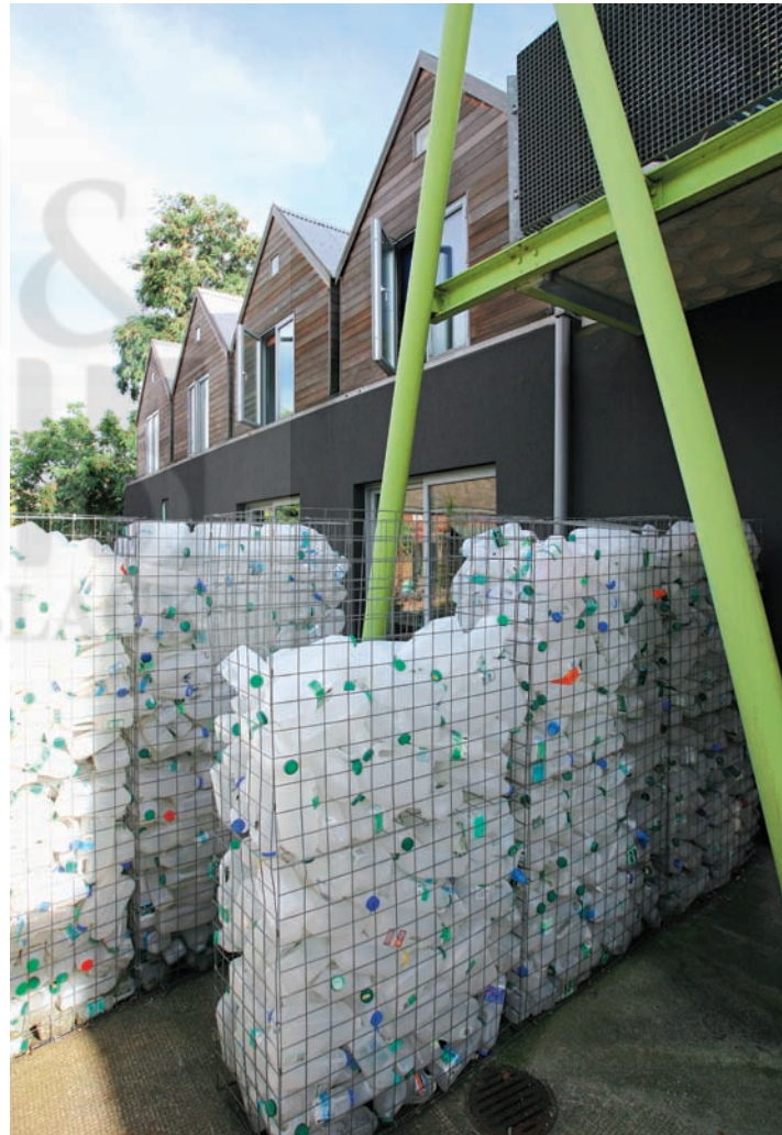
Milk Container Wall , Julia Manheim/Ken Taylor, 2006. Plastic milk containers, steel gabions. Photo: Anthony Coleman
