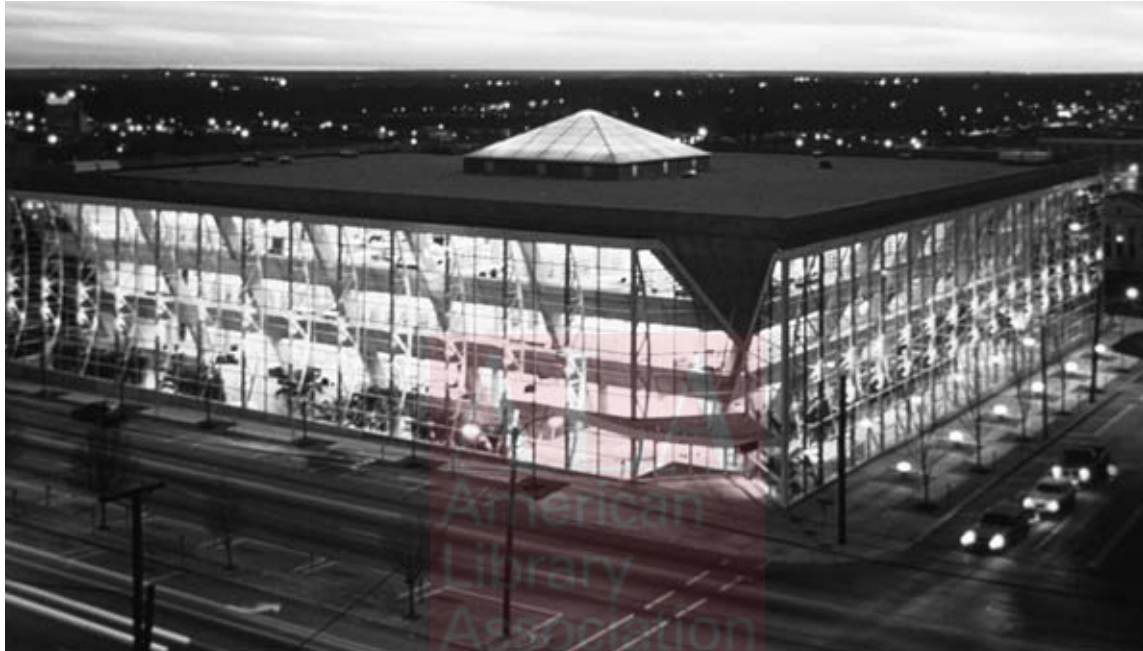
Exterior of library, Richland County Public Library, Columbia, S.C. Architect, Eugene Aubrey with Stevens and Wilkinson. Used by permission of the photographer.
