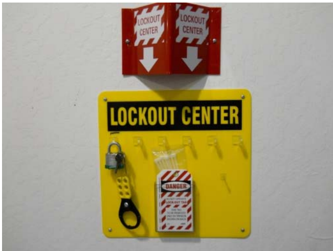
Figure 3.3. Example of a LOTO work station.
