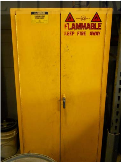
Figure 9.1. Closed flammable liquid storage with placarding.
