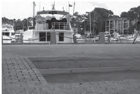
Fig. 22.1 Making the Harbor Accessible: A Ramp That Blends in With the Surroundings. (Photo by Janie B. Scott, August 20, 2011)
