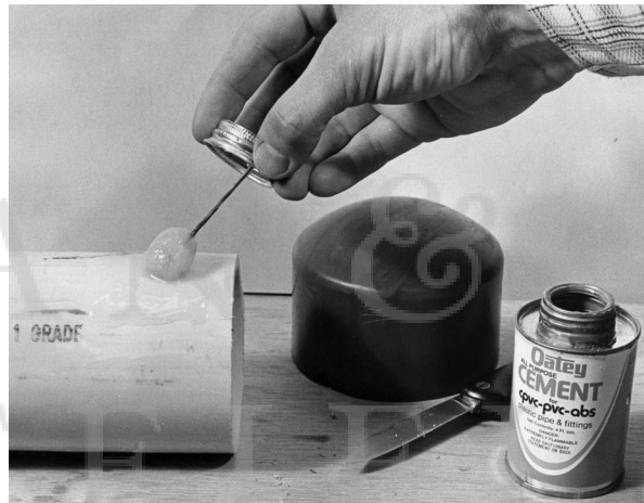
A second slip-on cap can be cemented to the other end using special PVC or other pipe cement.
