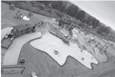
Figure 7.8 Playground areas in the UK have been surfaced using tyre crumb mixed with a PU binder. Reproduced with permission from the WRAP Quality Protocol, Waste and Resources Action Programme, Banbury, UK. ©WRAP (see note with Figure 7.1 )
