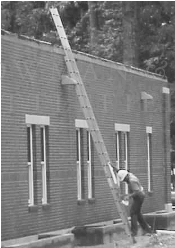
Figure 16-2. Ladder hazard
