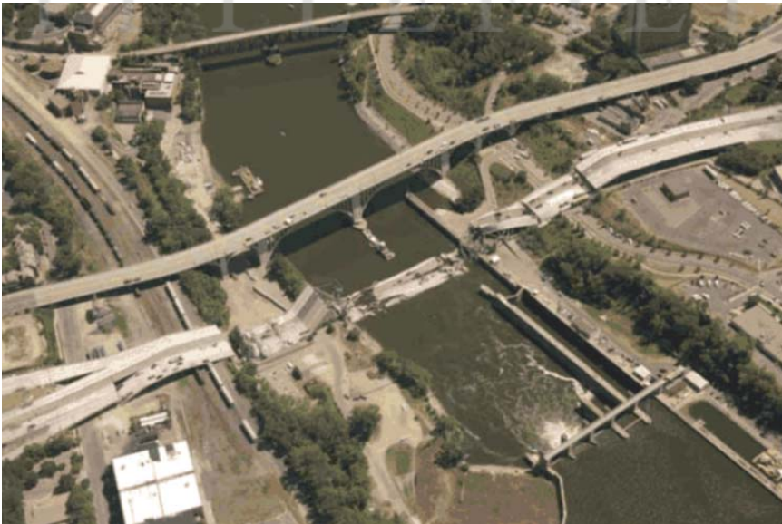
Photo 9-1. Minnesota bridge collapse (copied from National Transportation Safety Board [2008])
