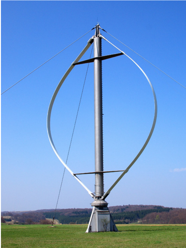
Figure 3.1. Darrieus rotor near Heroldstatt in Germany.
