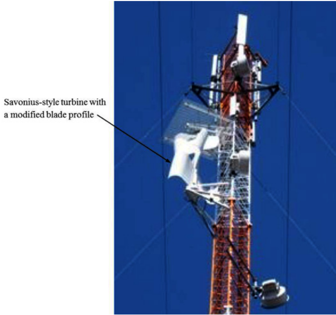
Figure 4.16. Application of Savonius-style wind turbines in communication towers with a modified blade profile.
