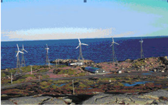
Figure 7.16. Small wind farm near the community of Ramea, Canada.
