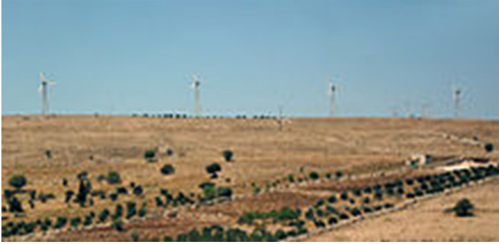
Figure 7.15. A view of Al-Ibrahimiya wind farm.
