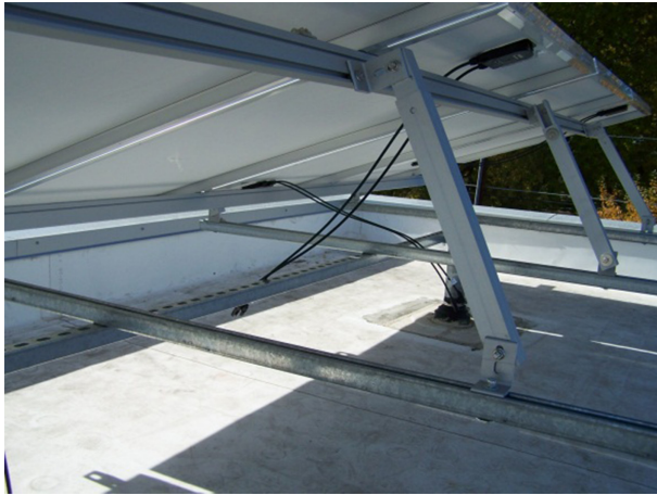
Figure 9.5. Tilt racking.
