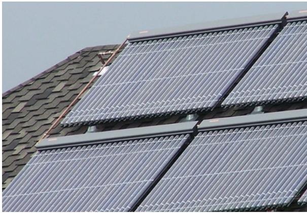
Figure 8.4. Vacuum tube collector.
