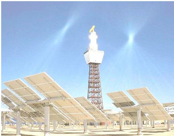
Figure 8.7. Solar thermal plant.
