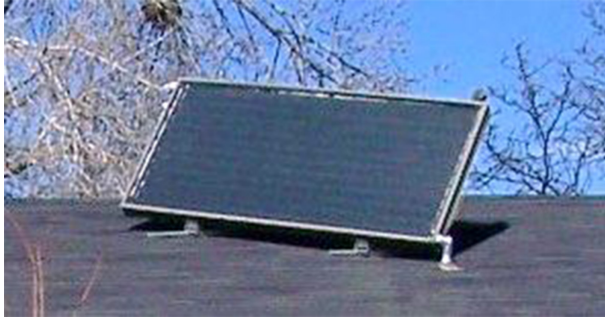
Figure 8.3. Flat-plate collector.
