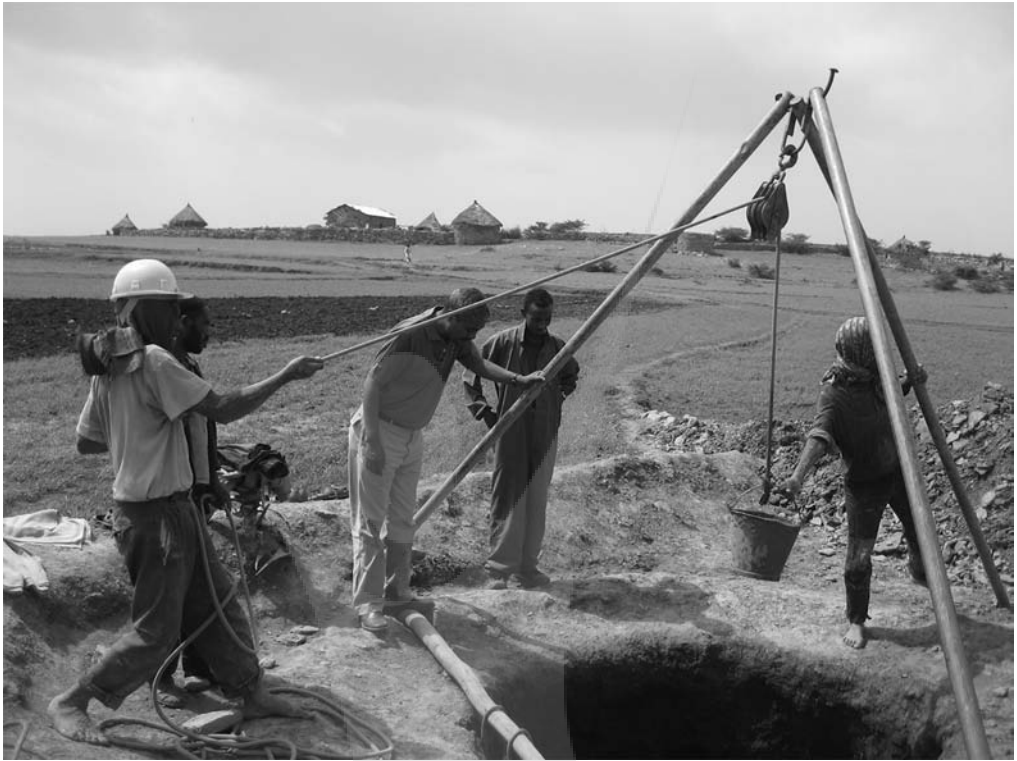
Digging the new well. Photo courtesy of water.org Flickr site.
