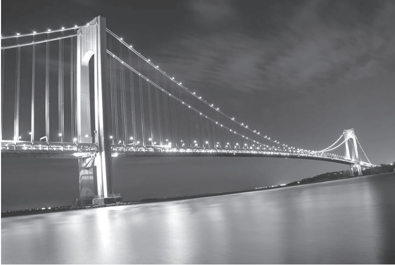
Figure 1.15 Verrazano-Narrows Bridge at Night from Brooklyn
