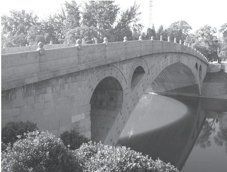
Figure 1.11 The Zhaozhou Bridge in China
