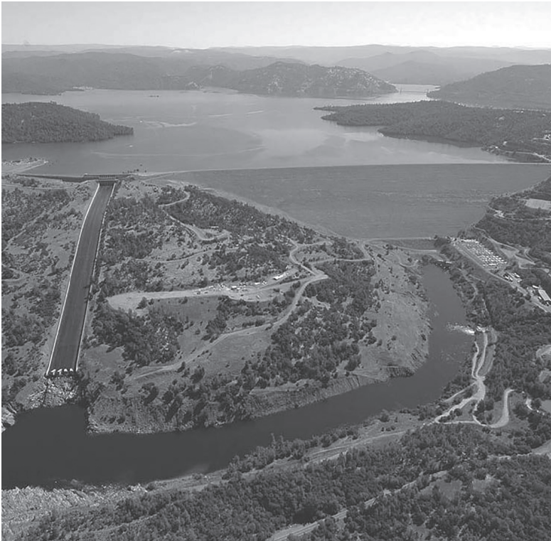
Figure 1.20 The Oroville Dam
