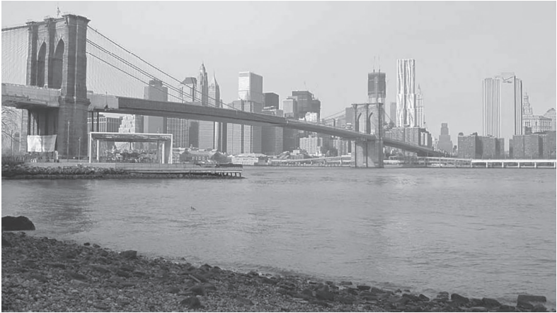
Figure 1.12 Brooklyn Bridge viewed from Brooklyn, with downtown Manhattan as a backdrop
