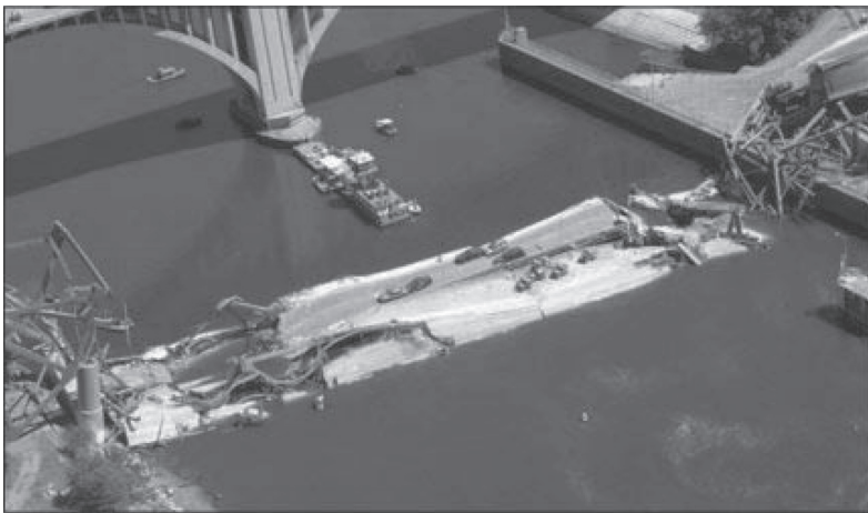
Figure 2.4 The collapsed main span of the I-35 W Bridge
