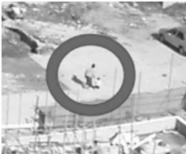
Figure 7.6 New Century Square construction site, Shanghai (2005)—detail
