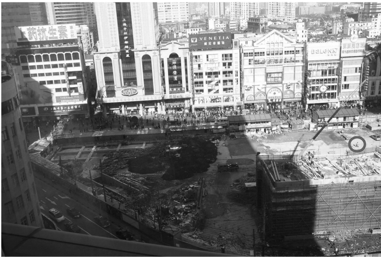
Figure 7.5 New Century Square construction site, Shanghai (2005)
