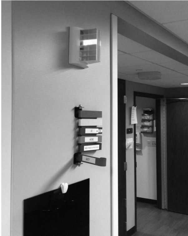
Figure 1.7 This image shows the manual flags with their surroundings and placement in the hallways. Above those is the light system that is used for visual management; each light has a meaning and can be seen from the central part of the hall (see Figure 1.3)
