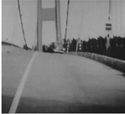
Figure 2.6. Torsion oscillations of the Tacoma Narrows Bridge.
