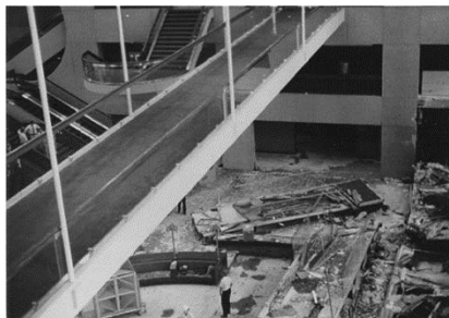
Figure I2.1. Hyatt Regency Walkway Collapse
