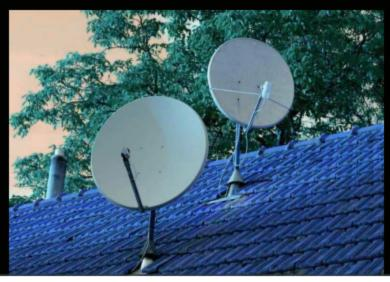
Satellite dishes receive digital signals directly from communication satellites. Satellite TV has a much larger range than broadcast TV, which transmits and receives signals using ground-based antennas.
