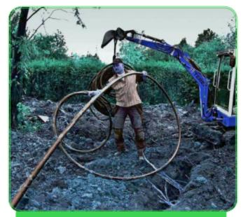
Pipes for a geothermal heating system are placed in the ground. The pipes help bring heat to a home.
