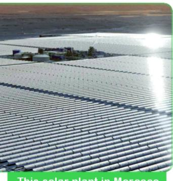
This solar plant in Morocco uses mirrors to collect energy from the sun. This is one of the world's largest solar plants. thermal solar plants, use mirrors to aim sunlight at pipes of water or oil. Water becomes steam as it heats up, while oil is used to make steam from water. The steam moves to a generator, where it turns a turbine. This makes electricity.
