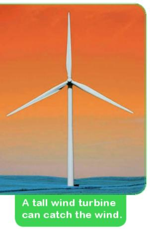
to charge our cell phones and devices, light our homes, and dry our clothes. How can the wind turn into electricity? Wind turbines are windmills that make electricity. We generate electricity by moving magnets around coils of wires. A wind turbine's job is to use the energy from the wind to move the magnets.
