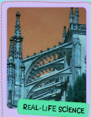
Builders and engineers working nearly a thousand years ago used the principle of the arch as they built great cathedrals. At first, they built thick buttresses against the outside walls. Then they realized that even the buttresses could be arch-shaped to do their job. Those supports are called flying buttresses.
