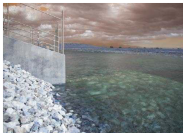
Arizona residents appreciate the water the CAP aqueduct brings.
