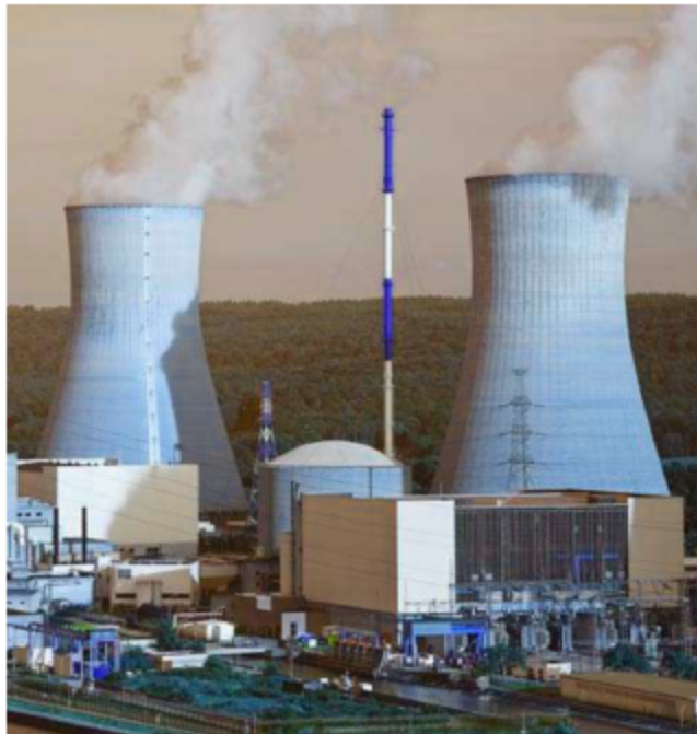
Water cools in giant towers at the nuclear power plant so it can be used again and again.
