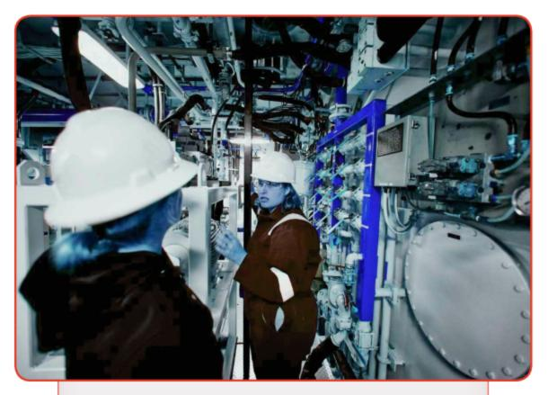
Mechanics must be familiar with every part of the systems that run huge ship engines, including electrical, piping, and wastewater. These are critical for the safety and comfort of the passengers and crew.
