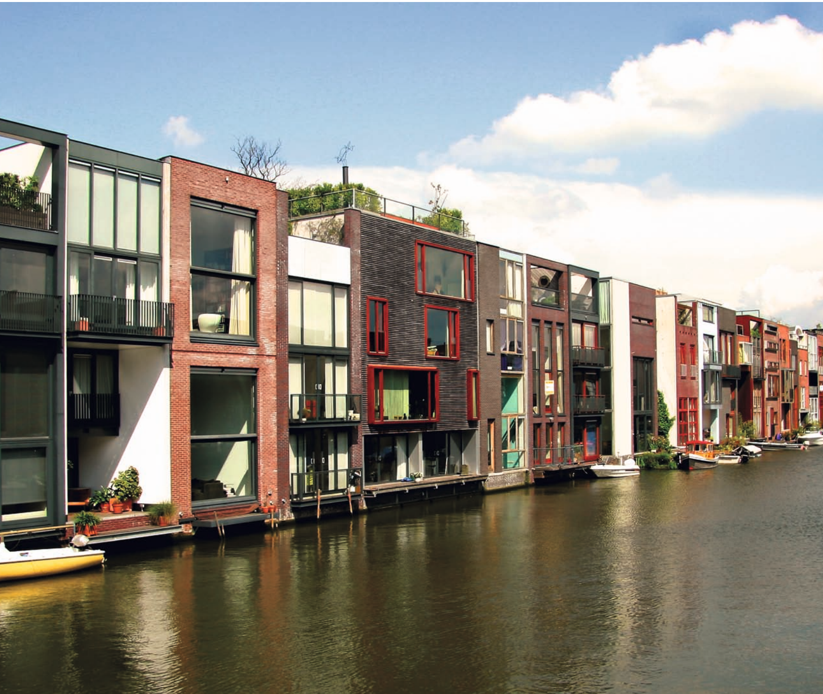
Figure 9.29 View of Borneo Sporenburg, masterplanned by West 8, taking a plot- based approach with each plot designed by a different team
