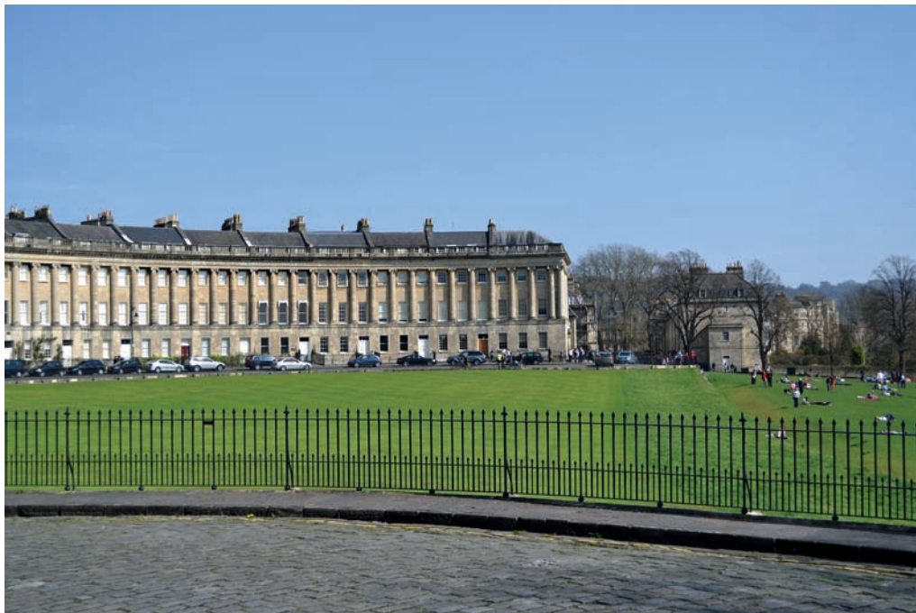
Figure 8.14-i View east across the green to the eastern side of the Royal Crescent and Brock Street
