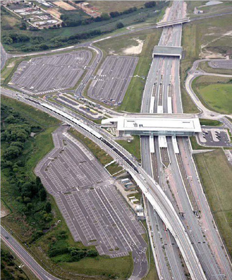
Ebbsfleet station and its new park-and-ride provision.
