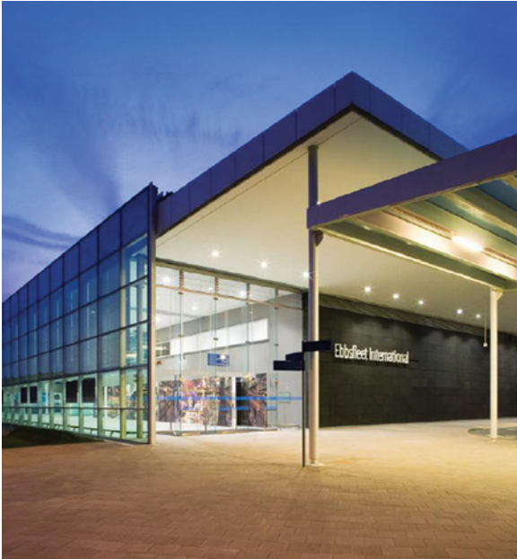
Ebbsfleet station entrance.
