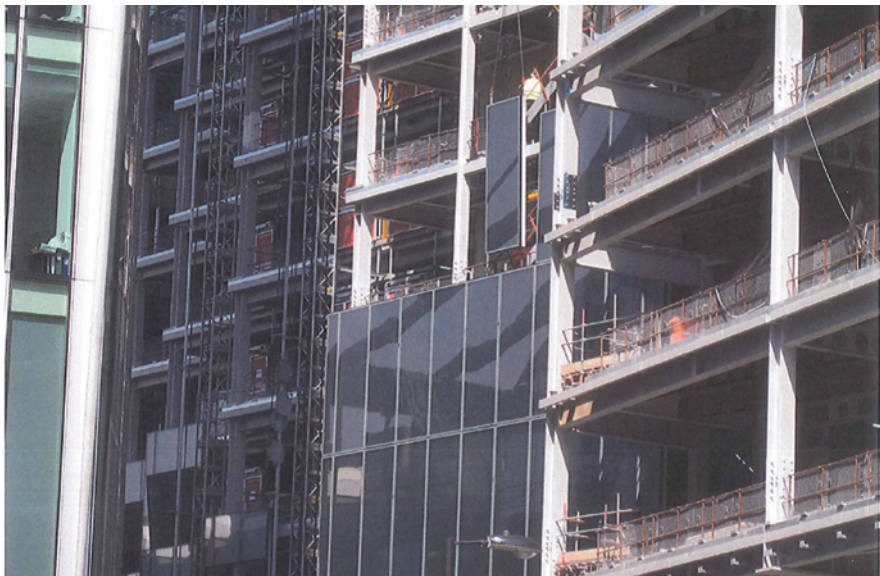
The façade panels being hoisted into place.
