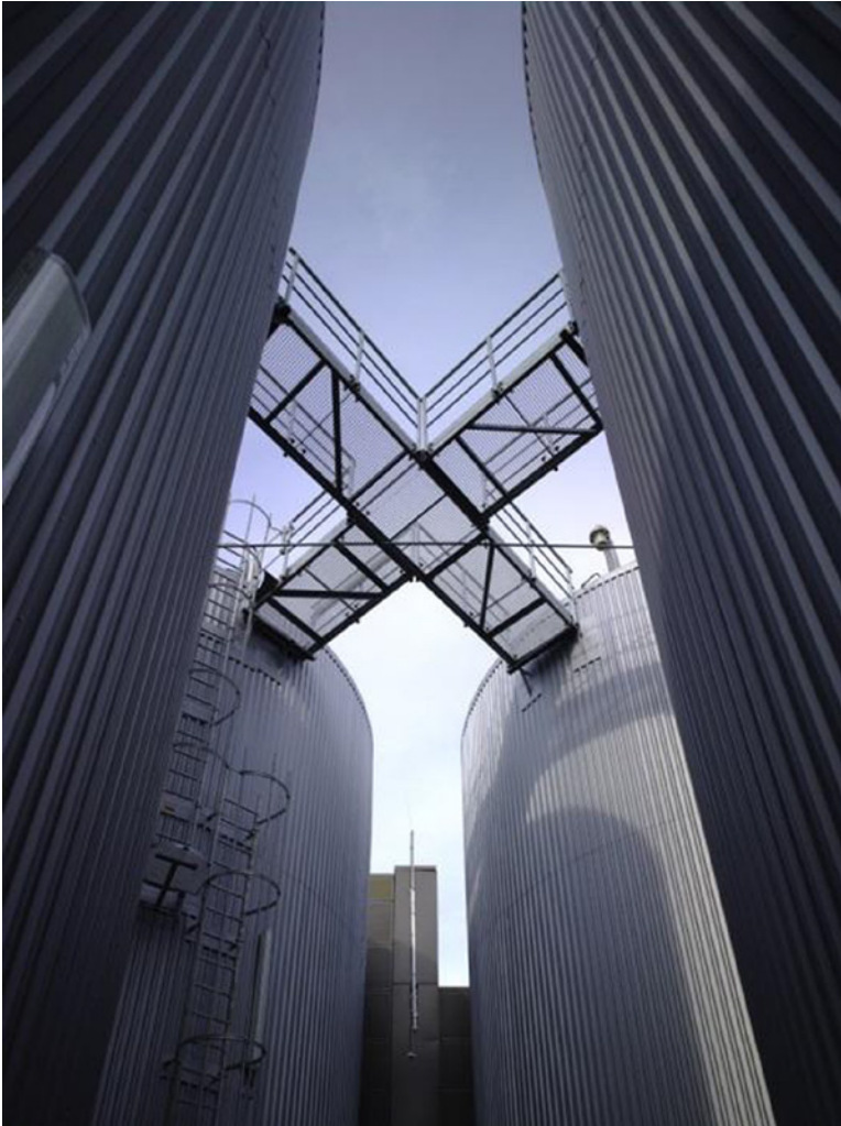
Cooling towers. Source: Image courtesy of Arup Associates.
