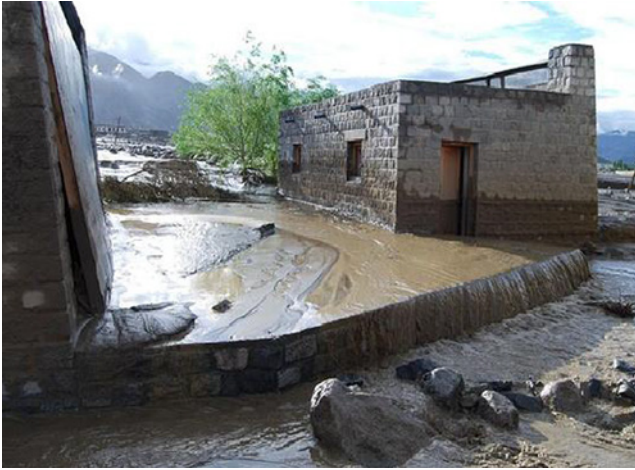
Aftermath of a mudslide in 2010.
