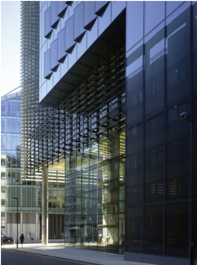
Main entrance south-east corner showing tilting windows.
