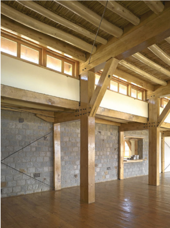
The finished timber structure.
