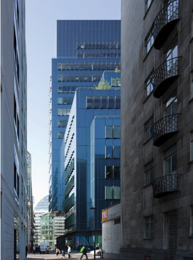
Ropemaker Place seen looking South along Finsbury Street.
