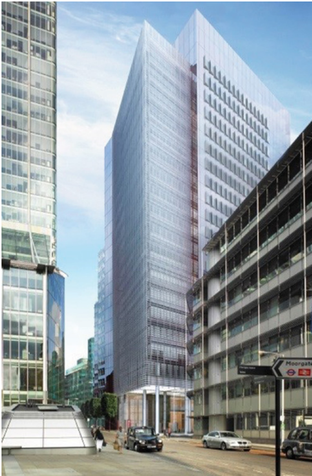
Ropemaker Place, London. Source: Image courtesy of Arup Associates.
