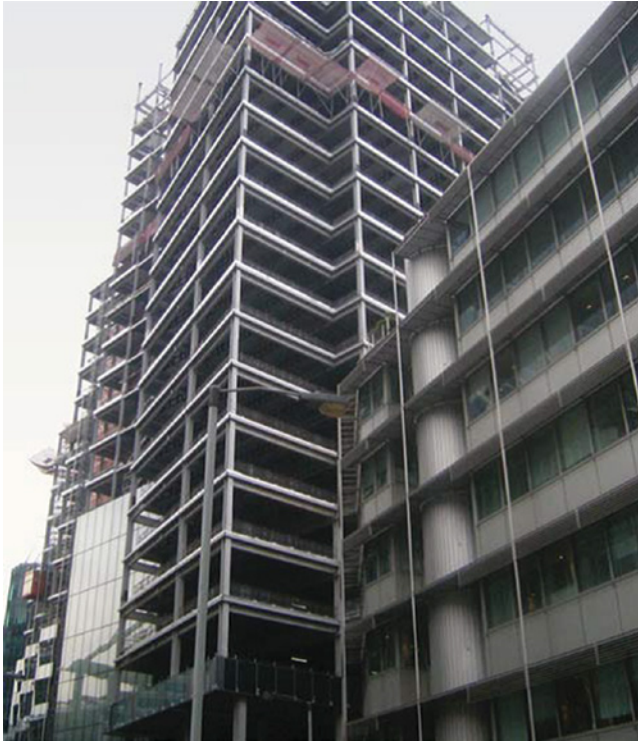
Steel frame nearing completion, and façade commenced.
