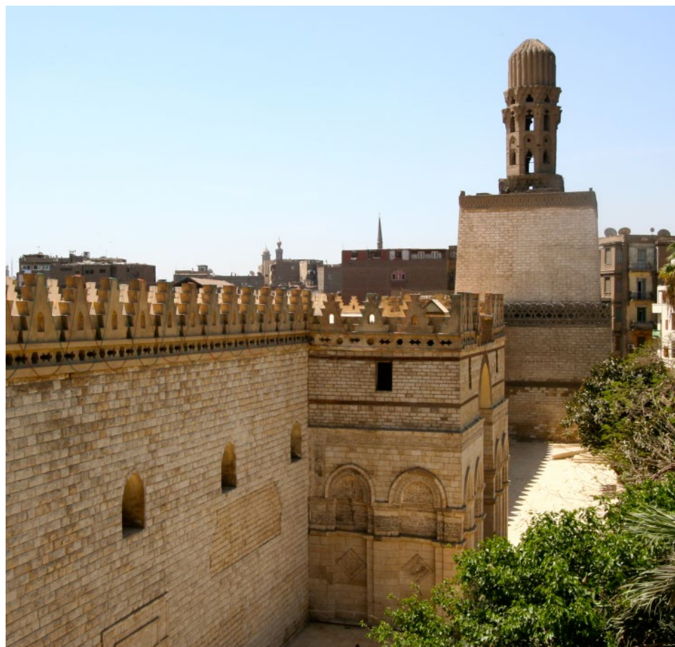
FIGURE 9.5 Mosque of al-Hakim, Cairo, south minaret with encasing, inscription, and reconstructed portal. Source: Jennifer Pruitt. Reproduced with permission.
