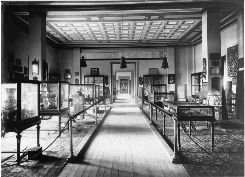
FIGURE 44.1 Installation of Islamic collections at the Ottoman Imperial Museum, Istanbul, 1891. “Müze-i Hümayun.” Source: Servet-i Fünun 984 (April 14, 1910): 348.
