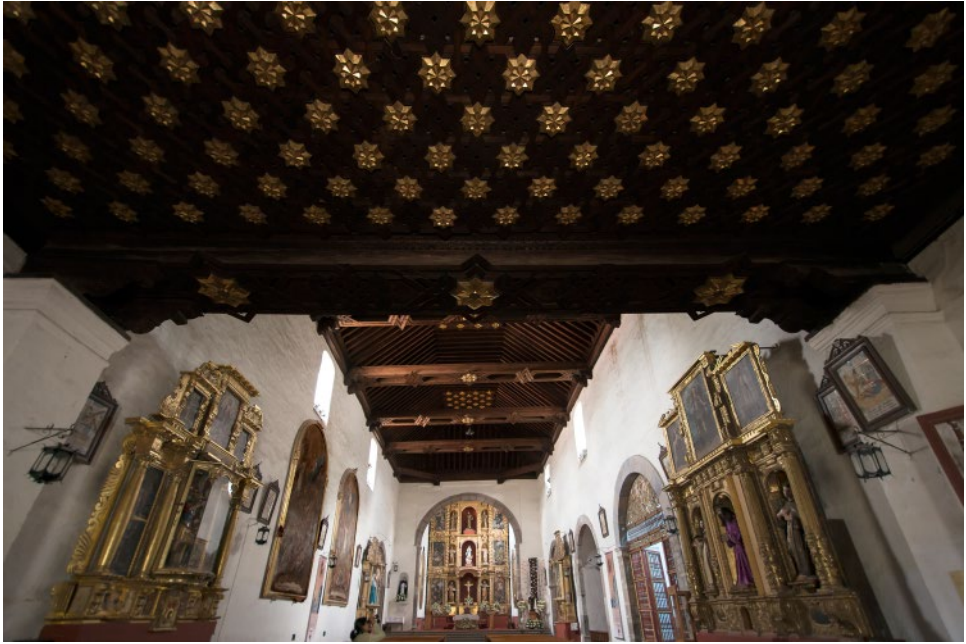
FIGURE 39.1 Artesonado at the Church of San Francisco in Tlaxcala, Mexico. Source: Eumelia Hernández. Reproduced with permission.
