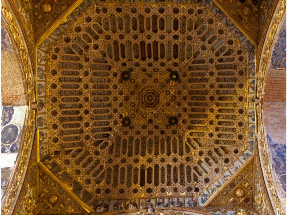
FIGURE 39.2 Artesonado at the Church of San Francisco in Quito, Ecuador. Source: Hernán L. Navarrete. Reproduced with permission.
