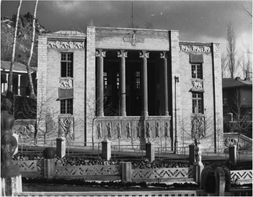
FIGURE 41.5 Front façade of the police prefecture ( shahrbani ) in Darband, northern Tehran, c. 1935. Source: Ali Khadem Collection, courtesy of Farrokh Khadem and Cyrus Samii. Reproduced with permission.
