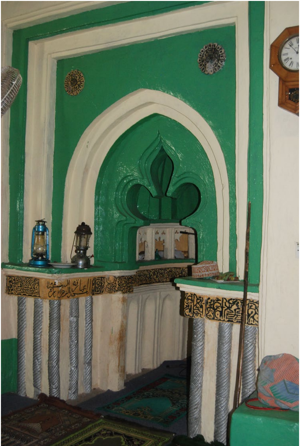
FIGURE 10.5 The mihrab at Kizimkazi, 1107. After its restoration, the coral was unfortunately covered in oil paint covering some of details of the carving and inscriptions. Source: Mark Horton. Reproduced with permission.
