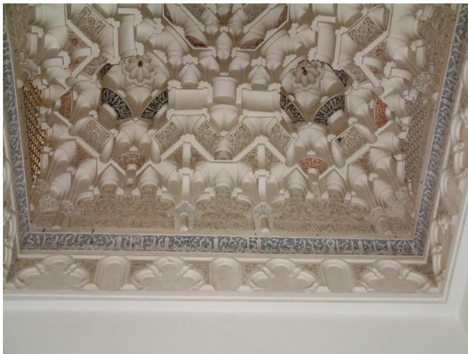
FIGURE 14.3 Rectangular muqarnas vault, al-Qarawiyyin Mosque, Fez. Source: Mariam Rosser-Owen. Reproduced with permission.
