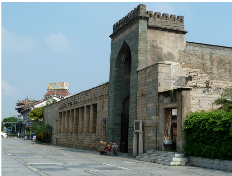
FIGURE 24.1 Entry and wall of Shengyousi, Quanzhou, 1009–1010; repaired 1310–1311. Source: Nancy Steinhardt.
