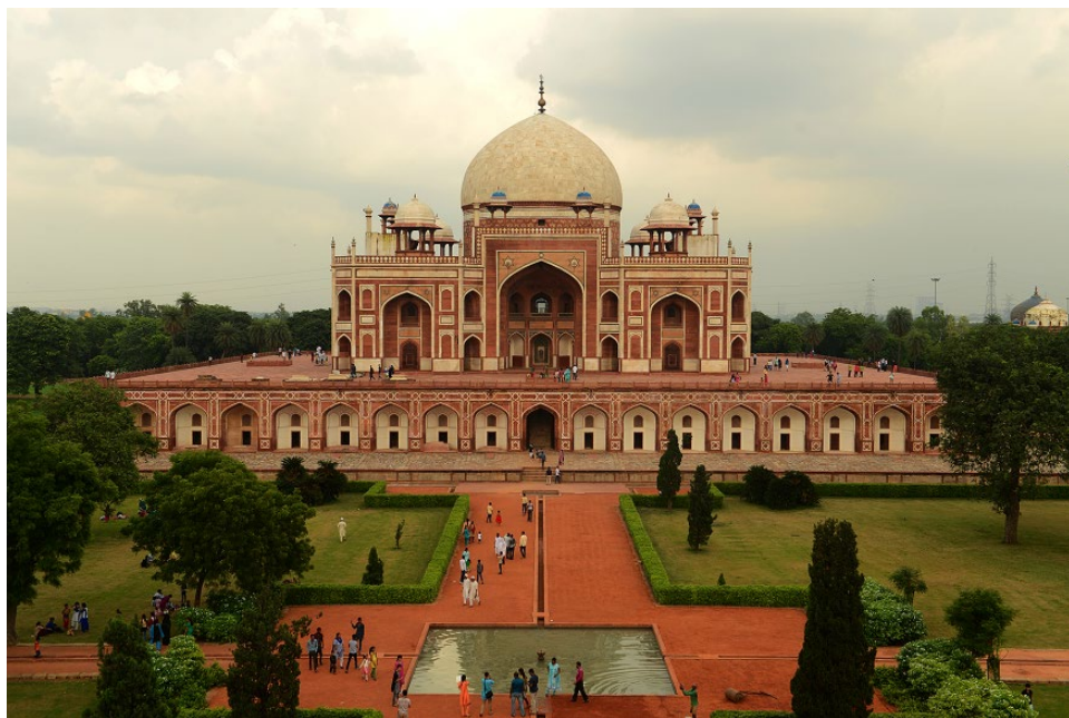
FIGURE 32.8 Tomb of Humayun after its restoration by the Aga Khan Trust for Culture, seen from the west. The restoration included the facing of the niches in the platform with white stucco plaster ( chunam ) and the renovation of the original tile mosaic of the small kiosks ( chhatris ) topping the frames of the grand entrance niches ( pishtaqs ). Source: Photograph by Narendra Swain, courtesy of Aga Khan Trust for Culture. Reproduced with permission.
