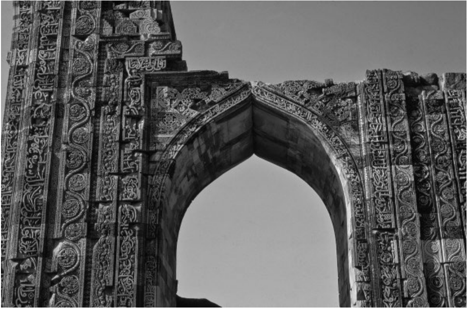
FIGURE 13.7 Detail of corbelled ogee arch of Qutb al-Din Aybak's screen showing vegetal and epigraphic borders, Qutb mosque, Delhi, c. 1200, showing Indic-style corbelled ogee arches and carved decoration of meandering vines, buds, and floral medallions. Source: Howard Crane. Reproduced with permission.
