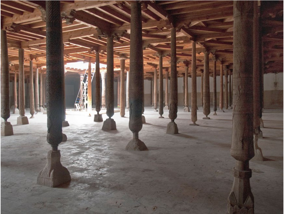
FIGURE 32.10 Jami' Masjid, Khiva, Uzbekistan, reconstructed in the eighteenth century with wooden columns dating from different periods reaching back to the ninth century and earlier. Source: Photograph by Britta Elsner, 2010. Reproduced with permission.
