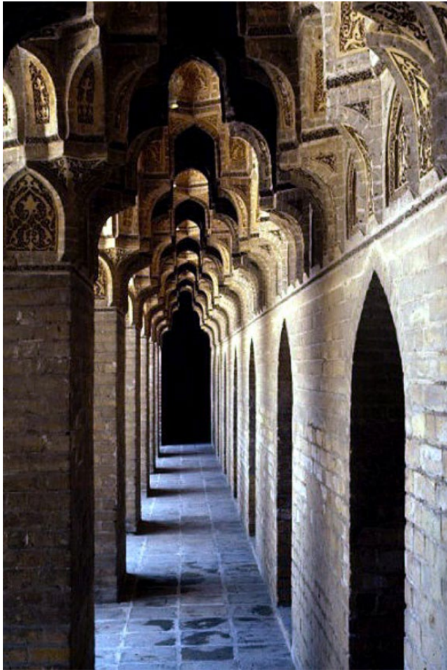
FIGURE 12.4 Baghdad: Abbasid Palace, c. 1200, corridor with muqarnas vaulting. Source: Yasser Tabbaa. Reproduced with permission.
