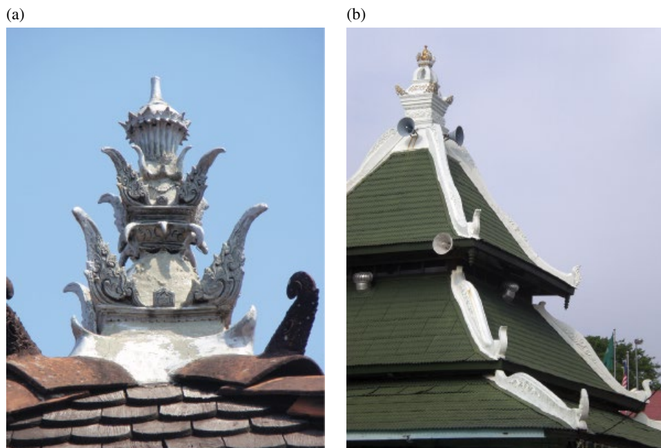
FIGURE 38.2 Roof ornaments and symbolism. (a) Memolo finial ornament from one of the pavilions in Kudus complex, Central Java. (b) Mustaka finial and Perabung Som ridge ornament, Pengkalan Rama mosque, Melaka.
