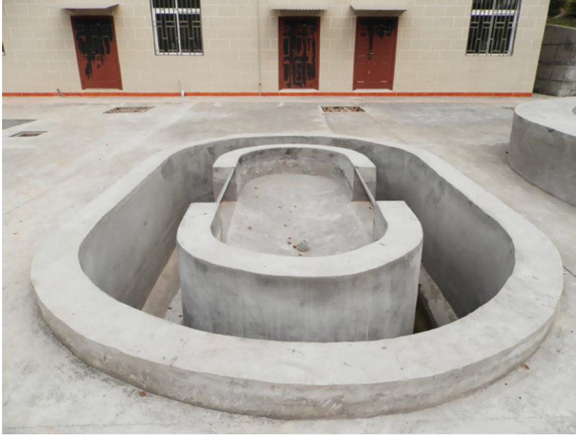
Figure 2.1.6 A concrete hatching tank used for incubation of grass carp eggs, popularly referred to as “Chinese Design of Concrete Hatching Tanks”, used for all major Chinese carp species. Source: Photo by Huihui Cheng.
