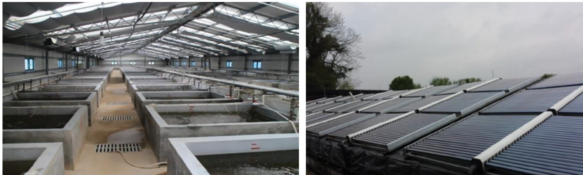
Figure 3.13.3 New greenhouse (left, light-shed plastic ceiling; right, shows solar energy heating equipment).
