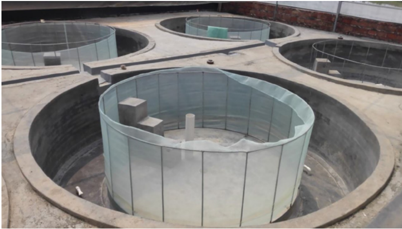
Figure 6.4.6 Circular incubating ponds (spawning pond of removable polythene nets and concrete stairs).
