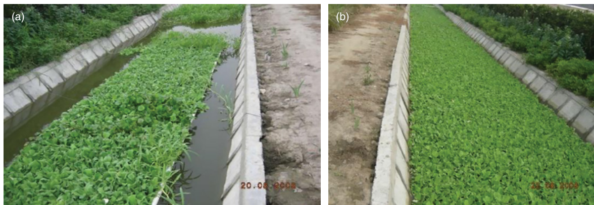
Figure 7.2.9 Examples of operational eco-channels: (a) compartmentalized on left; (b) non-compartmentalized on right.
