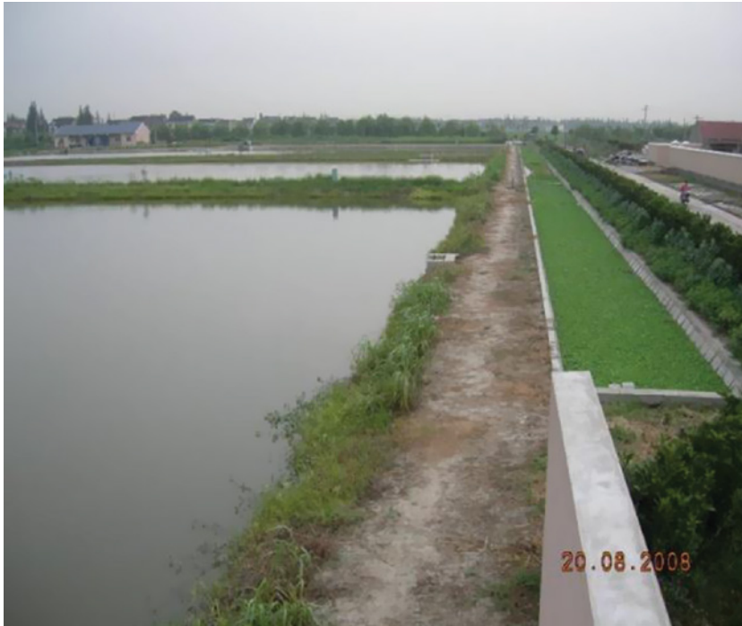
Figure 7.2.13 An operational pond recirculating aquaculture system.
