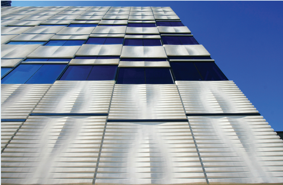
Figure 6-6 Detail view of precast and glass wall system Image courtesy of LMN Architects
