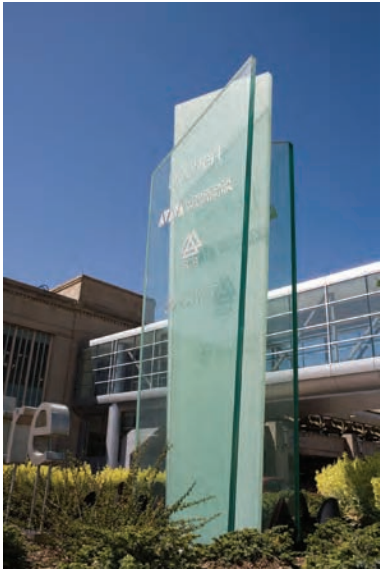
6.43 Three laminated glass panels comprise the tenant identification pylon at Philadelphia's Cira Centre. The middle panel uses a translucent lamination interlayer; the outside panels use an optically clear interlayer.
