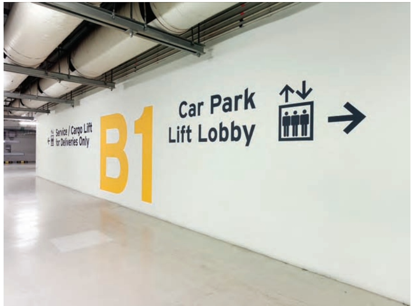
5.67 Frisket-painted graphics on a masonry wall provide durability and large-scale reproduction in a parking garage in Singapore.
