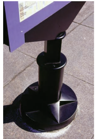
6.36 The federal star feature of this cast aluminum base distinctly brands all of the signs in Washington, DC’s citywide signage program. A north arrow cast into the base orients visitors to the City’s street plan.
