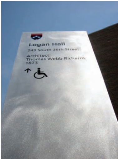
6.66 Random finish applied to aluminum panels provides visual interest and hides scratches on exterior signs at the University of Pennsylvania in Philadelphia.
