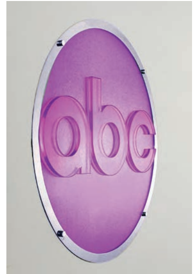
5.69 Solid cut glass letters laminated to a glass logo field at ABC Broadcasting's New York City headquarters.
