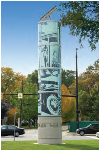
6.44 Curved glass panels are laminated with a printed translucent interlayer for the Woodward Avenue Tribute towers in Detroit. Interlayers can be printed in full color or black and white.
