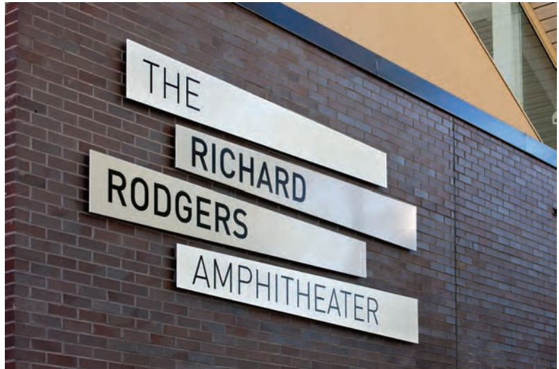
6.35 No waste: A single sheet of aluminum cut into wedge shapes and arranged in a staggered formation evokes music and rhythm for this Harlem, New York, amphitheater.
