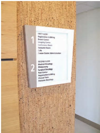
6.42 Clear acrylic directory sign with masked and painted areas that reveal a window for changeable information at a Stony Brook University medical building, New York.
