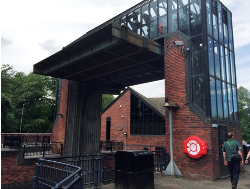
Figure 3.22 The Foss Flood Barrier in York, shown in the opened position to allow water to pass through (Source: Boshier, 2015).
