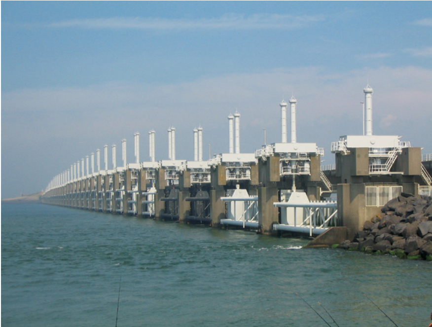
Figure 3.19 The Oosterscheldekering surge barrier, Netherlands (Source: Vladimír Šiman).
