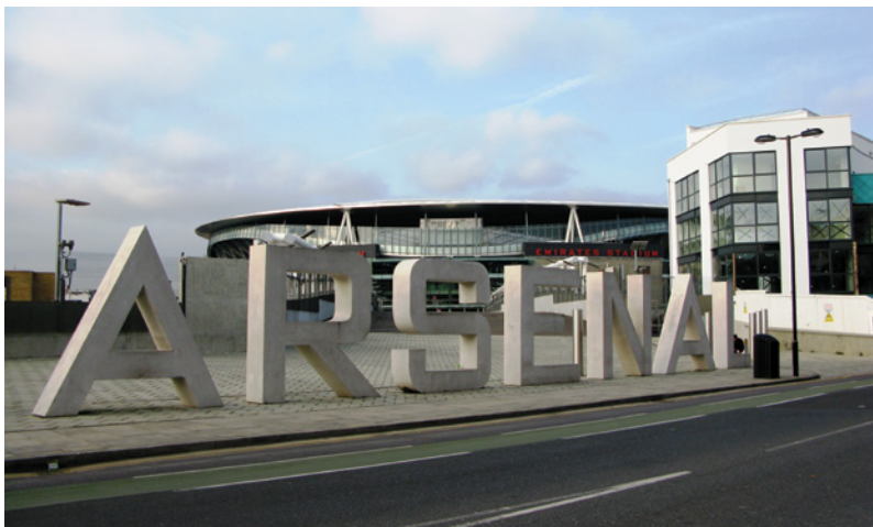
Figure 8.3 'Arsenal' sign used to restrict vehicular access to the Emirates Stadium, London (Source: Lee Boshier).
