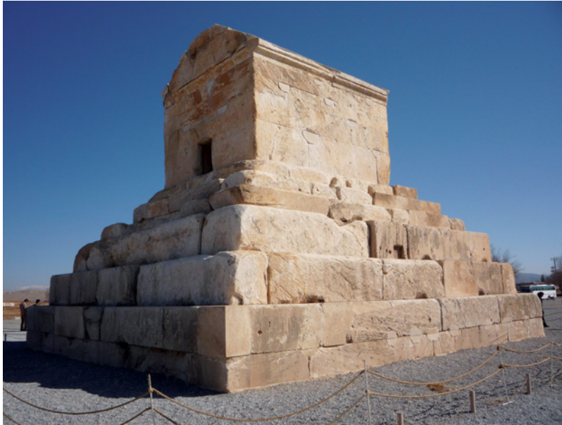
Figure 5.9 Tomb of Cyrus in Iran is said to be the oldest base-isolated structure in the world (Source: Reproduced with permission of Fahimeh Fotouhi).
