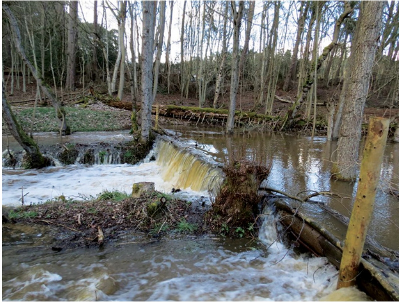
Figure 3.18 A woody debris dam used as part of an environmentally friendly and cost effective flood alleviation scheme on the upper catchment of the River Derwent, England (Source: Reproduced with the permission of Forestry Commission).
