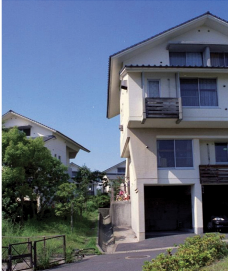
Figure 6.12 An example of urban design used to mitigate the effects of ash fall in Kagoshima, Japan. The design of the housing includes gutter-free roofs (which have a storm water channel located directly beneath), ash-resistant tiles, heavy-duty rubber window and door seals (to aid air tightness to prevent ash entering houses) and large overhanging roofs over balconies ( Source : Reproduced with permission of David Johnston).
