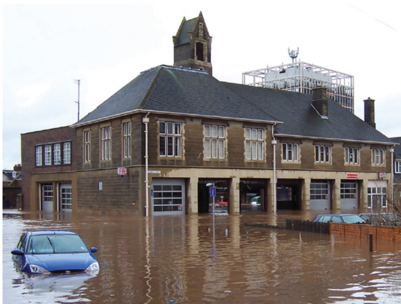
Figure 3.3 Flooding in Carlisle, England in January 2005. Poor planning contributed to critical services such as the emergency services, local government offices and electricity substations being located in flood prone areas (Source: © ICDDS).
