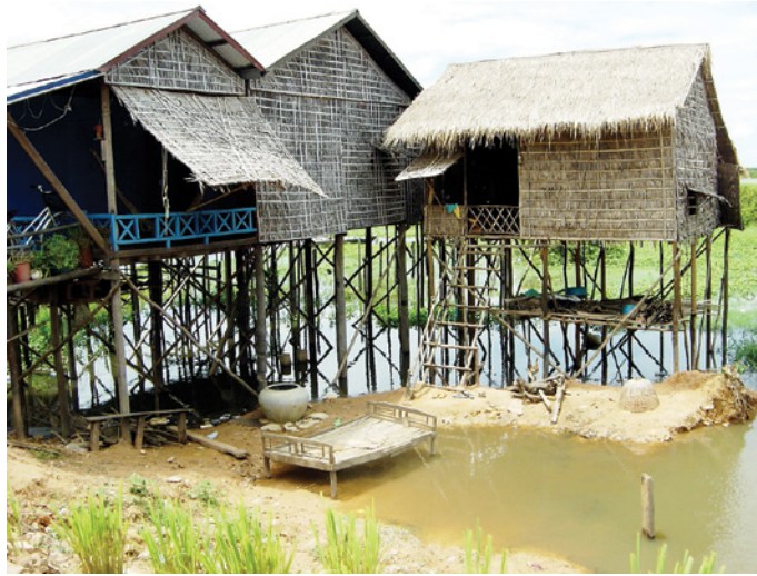
Figure 3.8 Traditional house elevated over a floodplain in Cambodia (Source: Reproduced with permission of Southopia on Flickr).
