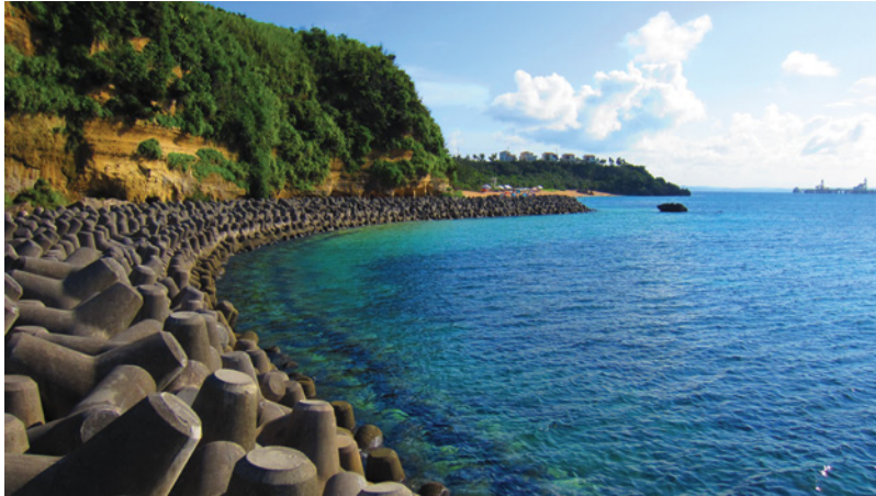
Figure 8.4 An example of concrete ‘tetrapods’ used to reinforce the coastline on Ikei Island, Japan (Source: Nelo Hotsuma on Flickr).
