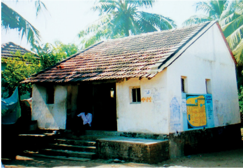
Figure 4.8 Traditional high status house in coastal area of Sri Potti Sri Ramulu, Nellore District of Andhra Pradesh, India. The house is built on an elevated plinth to protect the property from localised flooding caused by storm surges (Source: Boshier, 2002).
