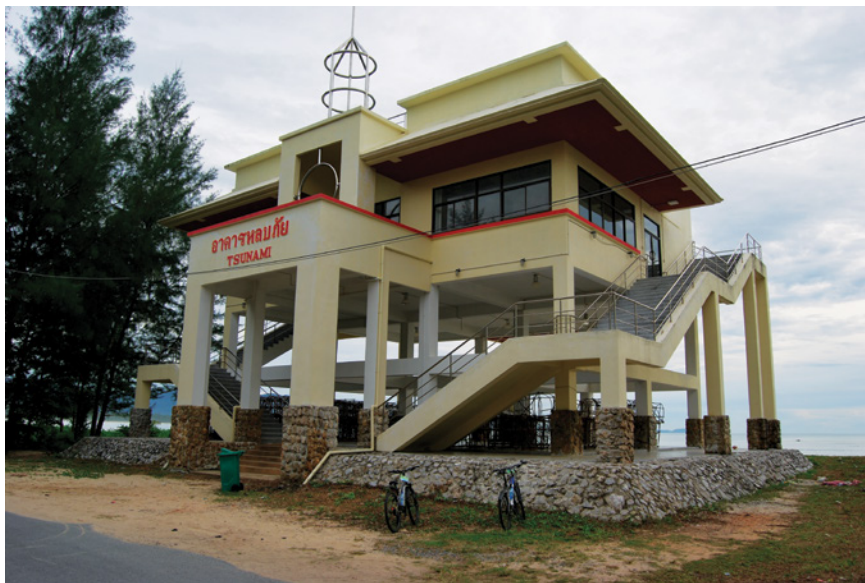
Figure 5.16 Tsunami shelter in Khao Lak, Thailand (Source: Roy Googin).
