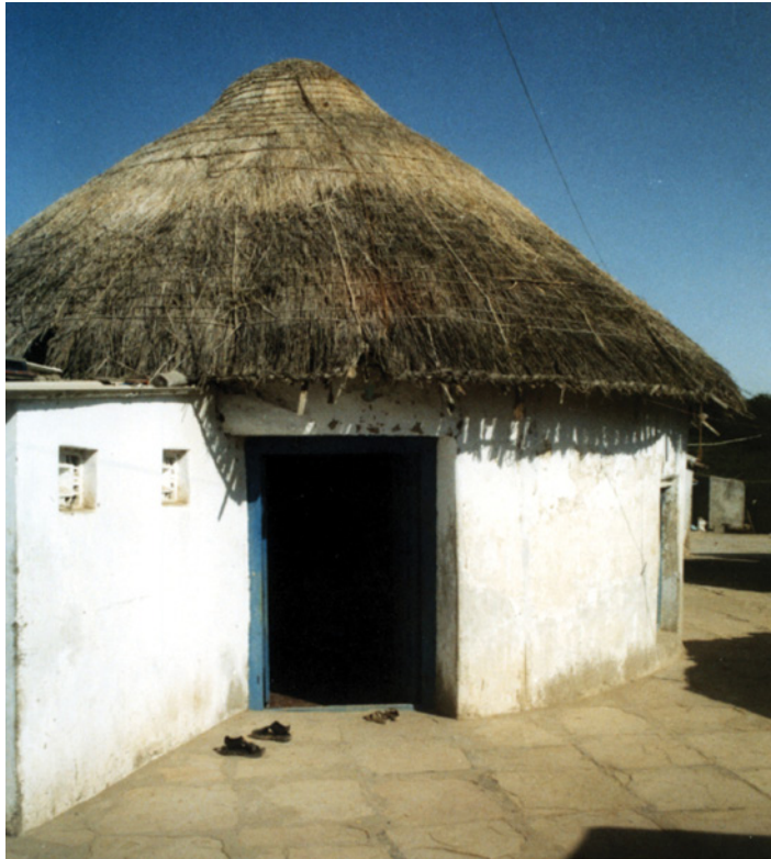
Figure 5.11 Bungla style house in a village near Bhuj in Gujarat, India (Source: Reproduced with permission of Matthias Beckh 2001).
