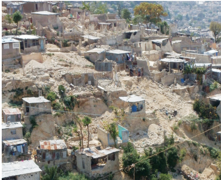
Figure 5.2 Extensive damage to housing caused by the Haitian earthquake in 2010 (Source: WEDC).
