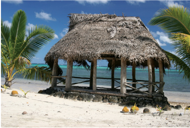
Figure 4.6 Typical fale'o beach fale, Manono Island, Samoa (Source: Reproduced with permission of Sonja Pieper).
