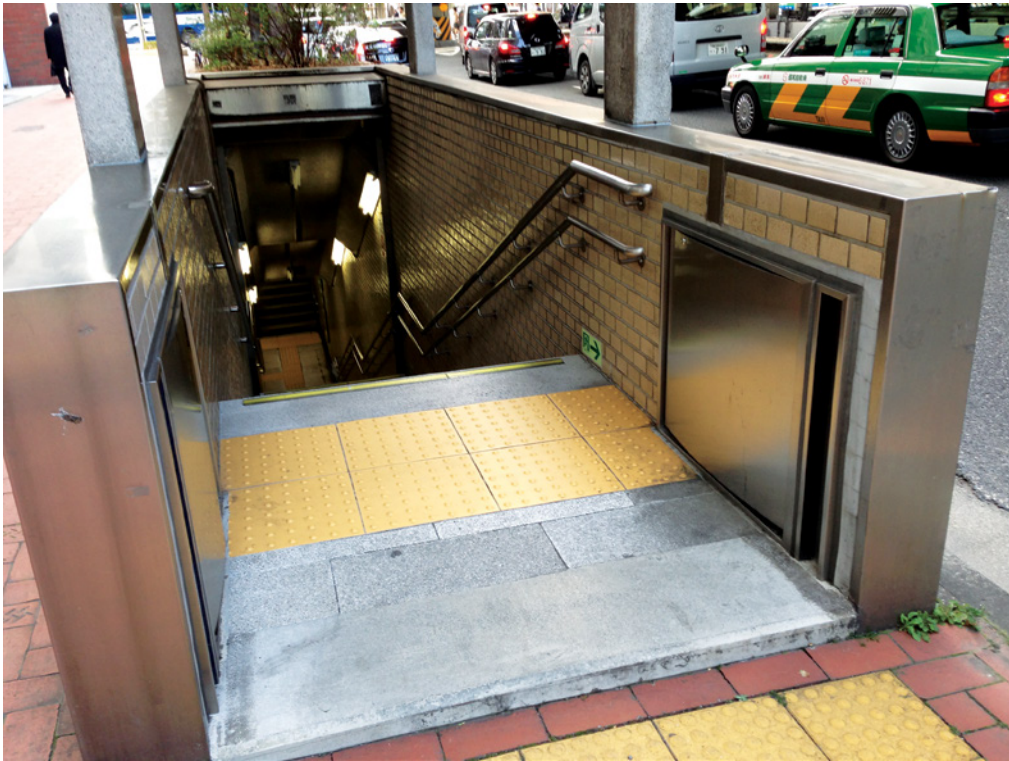
Figure 3.25 Flood gates at an entrance to the Tokyo Metro system. These barriers can be deployed quickly to protect the Metro system in the event of a potential flood (Source: Boshier, 2015).
