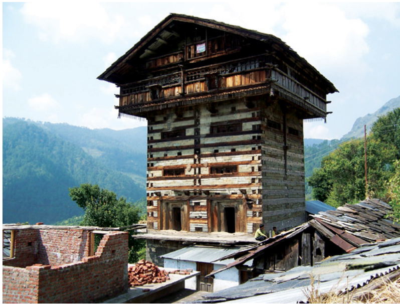
Figure 5.14 Example of a Koti Banal (timber reinforced masonry) building in Northern India (Source: Reproduced with permission of Dominik Lang).
