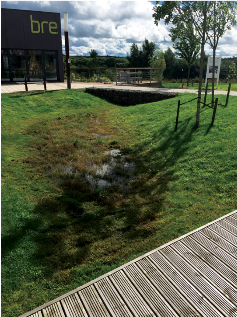
Figure 3.21 SUDS in use at the Building Research Establishment's Innovation Park (Scotland): Examples of swales and permeable paving (Source: Boshier, 2015).
