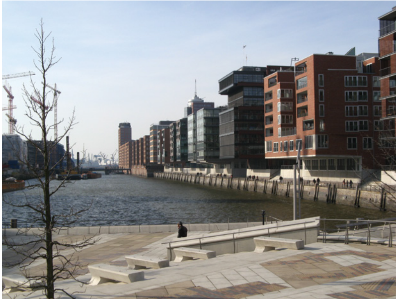
Figure 8.6 Hafencity: Utilising a masterplan that considers the interaction between existing and new buildings, the waterfront and the elevation of buildings as a flood protection concept (Source: Reproduced with permission of M. Pinke on Flickr).
