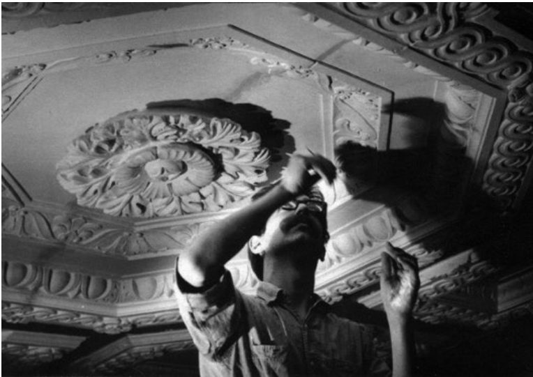
Figure 7 Author installing an ornamental plaster ceiling, Wilkes Barre, Pennsylvania, while employed at Felber Studios, Horsham, Pennsylvania. 1970. Source: Photograph courtesy of author’s archives.
