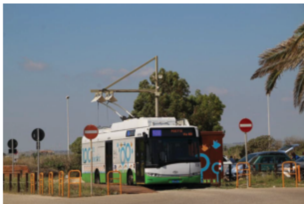
Fig. 4.10. Station for stationary charging of trolleybuses, Cagliari, Italy
