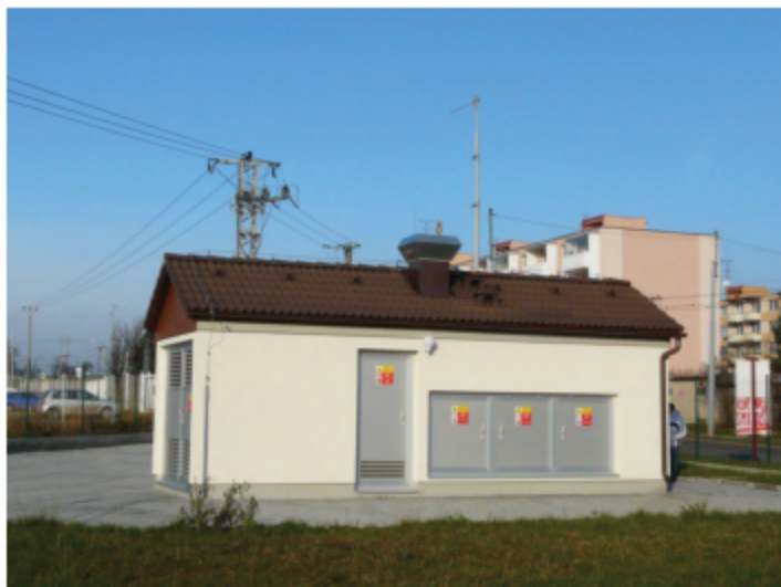
Fig. 4.12. Compact trolleybus substation, Bmo, Czech Republic
