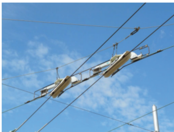
Fig. 4.8. High speed crossing of the tram and trolleybus overhead line, Ostrava, Czech Republic
