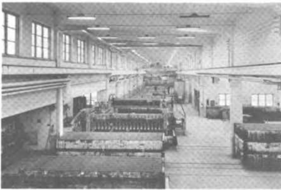
Fig. 1 - Swedish factory for making autoclaved cement-silica cellular concrete showing multi-level form cars with uncured material cut into slabs and blocks.
