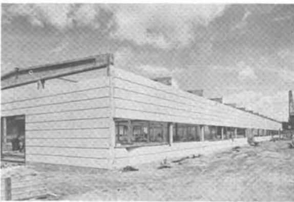
Fig. 3 - Partially completed factory building with walls of autoclaved cellular concrete.
