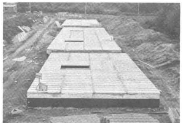
Fig. 4 - Floors of houses made of autoclaved cellular concrete.
