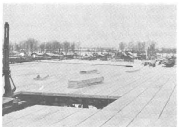
Fig. 6 - Roof construction with autoclaved cellular concrete for factory building.
