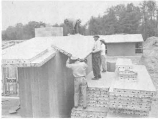
Fig. 7. Stressed skin panels used in a cathedral ceiling
