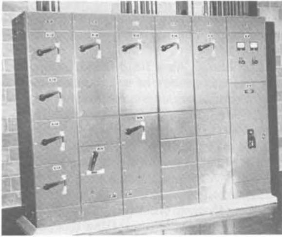
Fig. 1. Typical motor control center.
