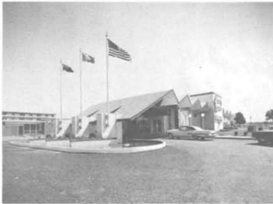
Fig. 9. Glued folded plate roof
