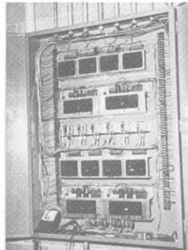
Fig. 4. Typical subtemperature control panel.
