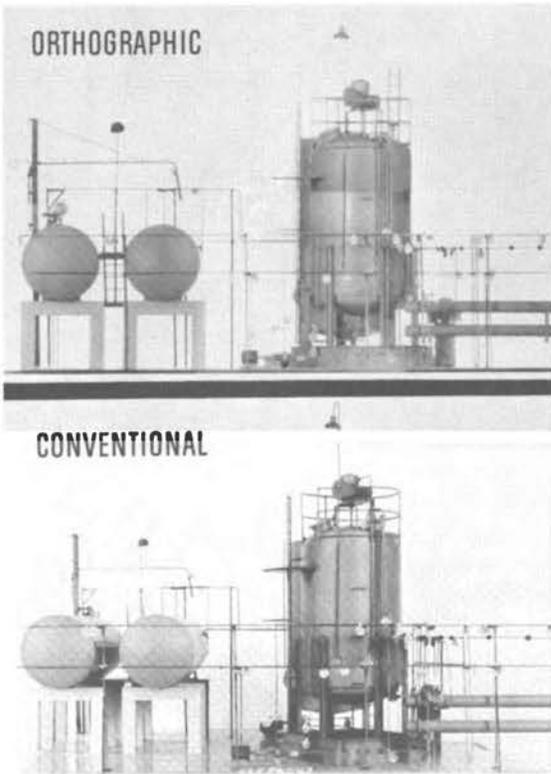
Fig. 9. Comparison of model photographs taken with a conventional camera (bottom) and with a non-perspective (orthographic) device.
