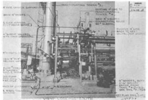
Fig. 10. Typical completed piping photo-drawing for a revision to an existing facility.
