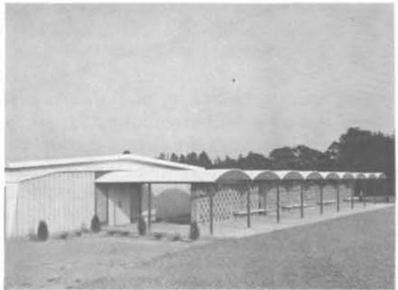
Fig. 10. Curved plywood panels form canopy
