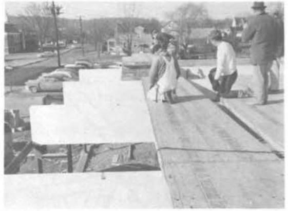
Fig. 8. Box beam - stressed skin panel roof system
