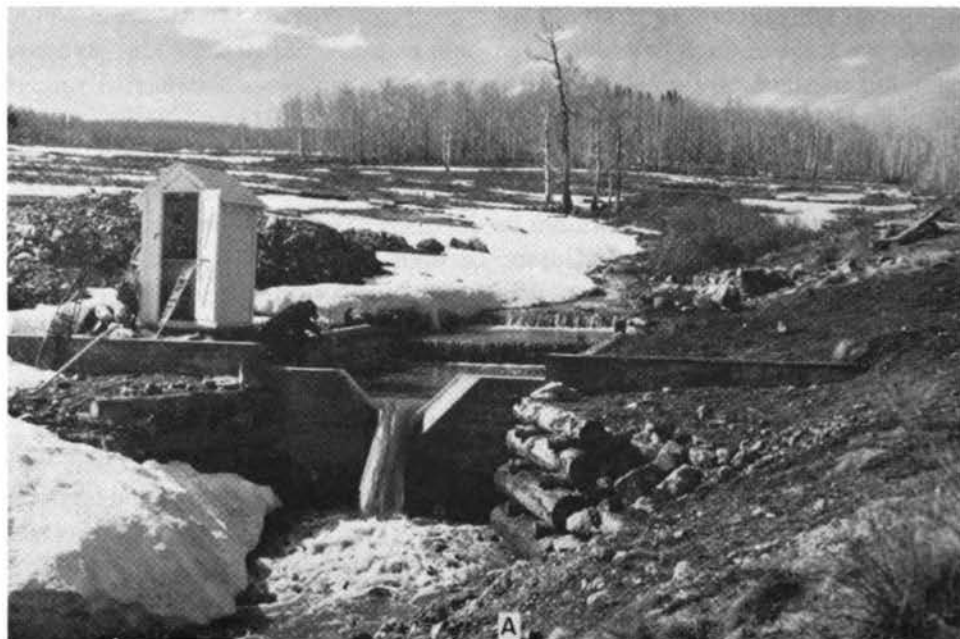
FIGURE 8. Four types of stream gauges. A , 90-degree, sharp-crested weir suitable for measuring small flows accurately where low temperatures are expected. B , One-foot San Dimas flume suited to passing sediment-laden flows. C , Trapezoidal flume suited
