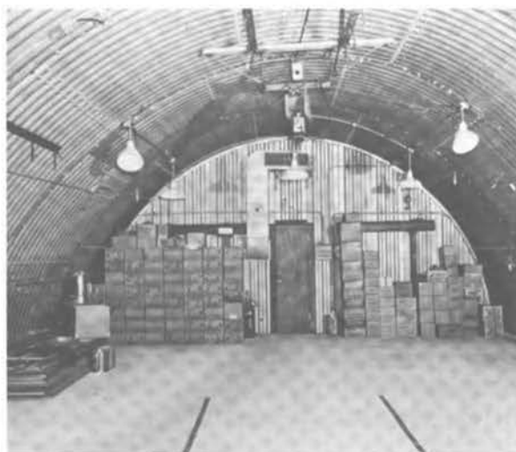
Figure 14. Interior view of shelter showing supply duct and grille
