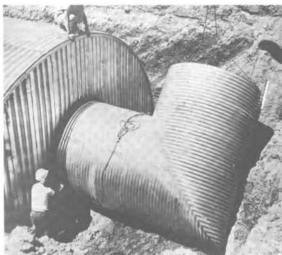
Figure 13. Exterior view of one end and entrance passage to the 100-man metal shelter
