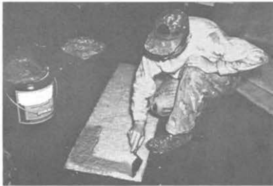
Figure 3. Pointing trowel used to apply adhesive on small insulation job.
