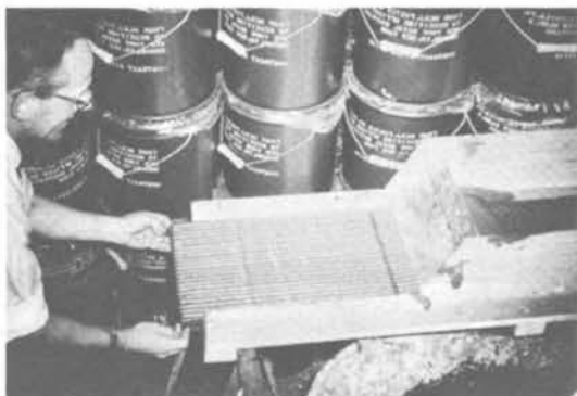
Figure 5. Push-box application of adhesive on cellular glass insulation.
