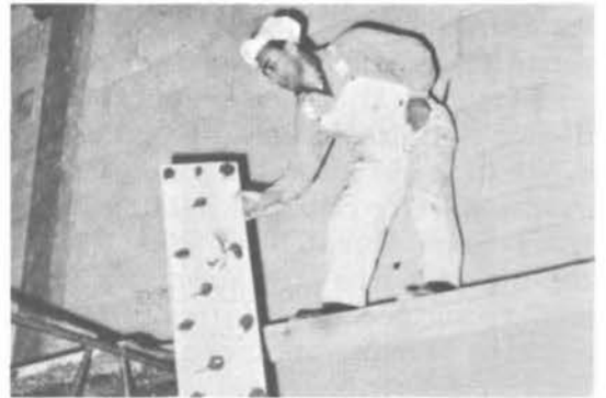
Figure 4. Gob application of adhesive on polystyrene foam for cooler-room insulation.
