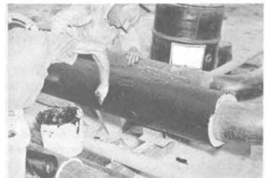
Figure 6. Bare-hand application of mastic adhesive on polyurethane foam pipe covering.
