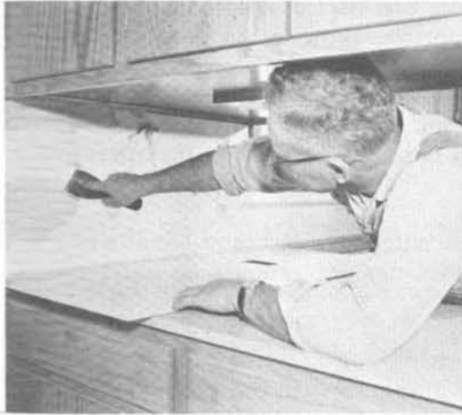
Figure 6. Application of mastics
