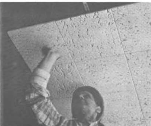
Figure 5. Final adjustment by hand pressure for leveling and setting.
