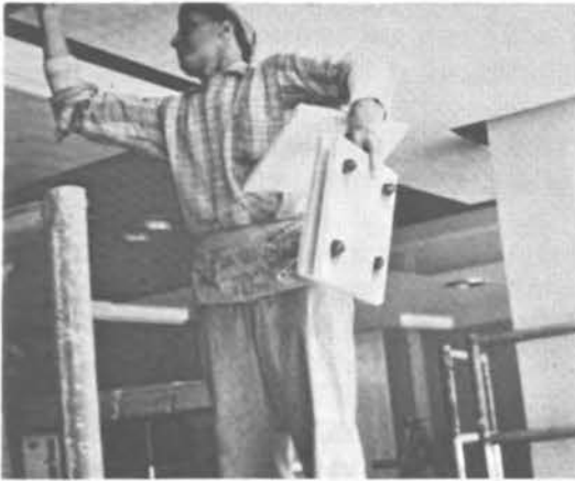
Figure 1. Four pats of adhesive properly placed.
