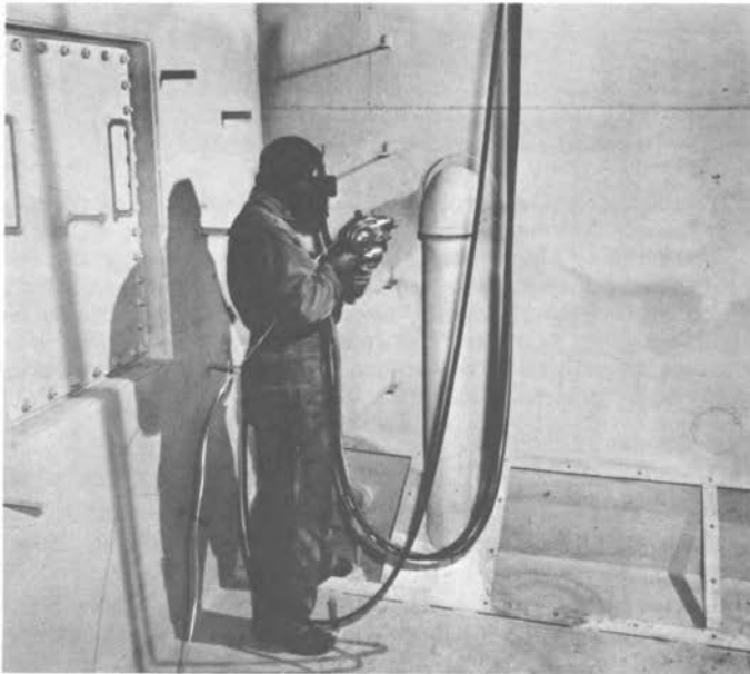
Figure 1--Metallizing operation shows tank being aluminumized to prevent corrosion.
