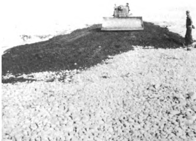
Fig. 3. Bulldozers spreading and compacting fill
