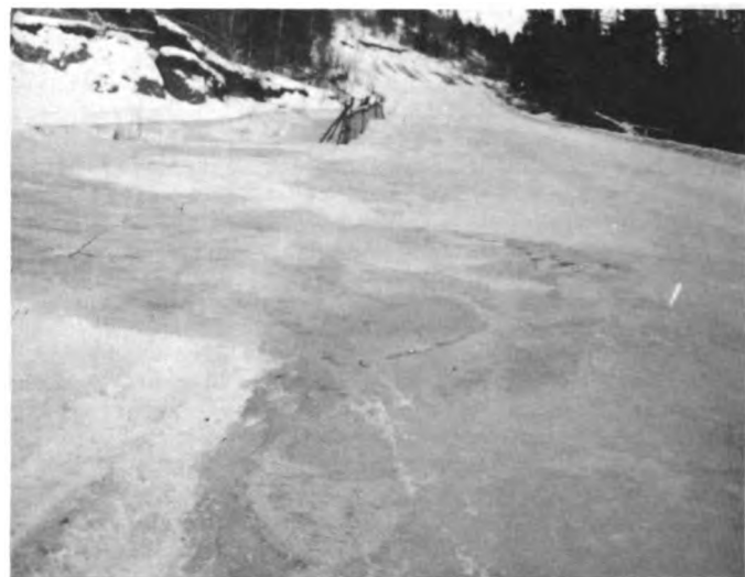
Fig. 1. Encroachment of ice on the road
