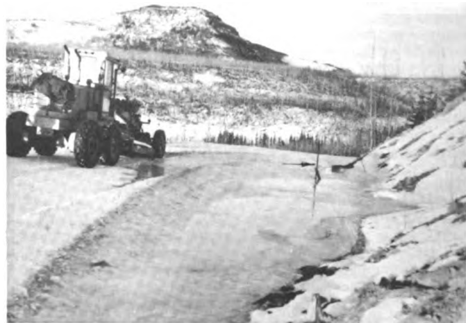
Fig. 7. Removal of ice from the road
