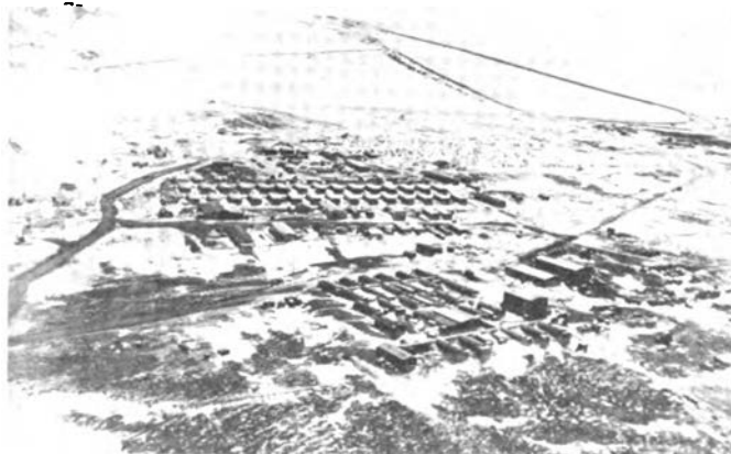
Fig. 1. Camp Tuto and roads on ice and permafrost (U. S. Army photograph)
