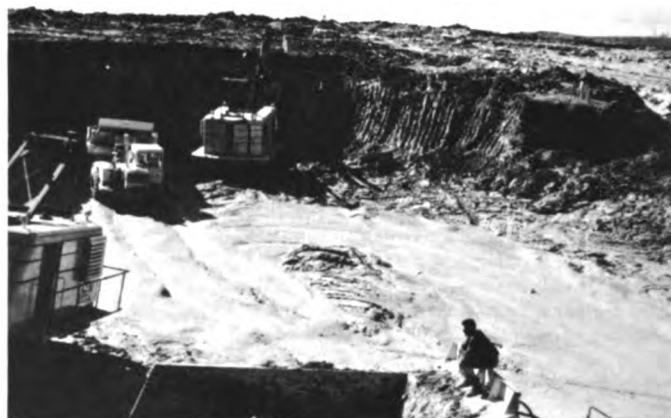
Fig. 3. Sluiceway excavation through overburden containing permafrost, August 1957
