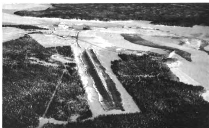
Fig. 8. Construction of No. 2 west, January 1959
