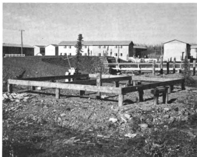
Fig. 4. Pile foundations for house
