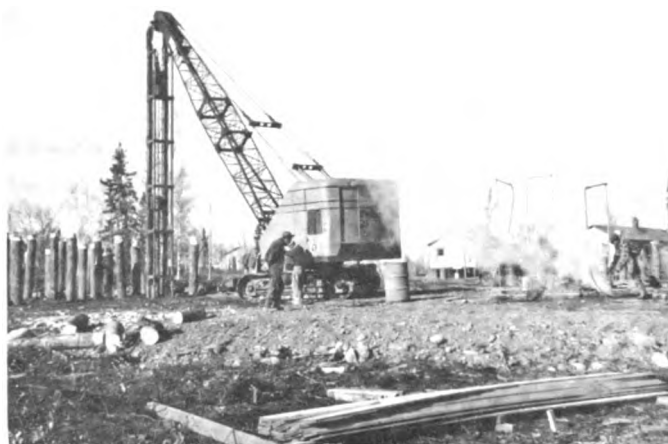
Fig. 7. Pile steaming and driving
