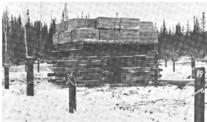
Fig. 2. Pile load tests in Site C, Fairbanks, Alaska
