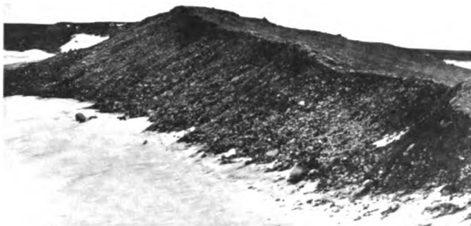
Fig. 4. View of original ramp road showing ablation effects (U. S. Army photograph)
