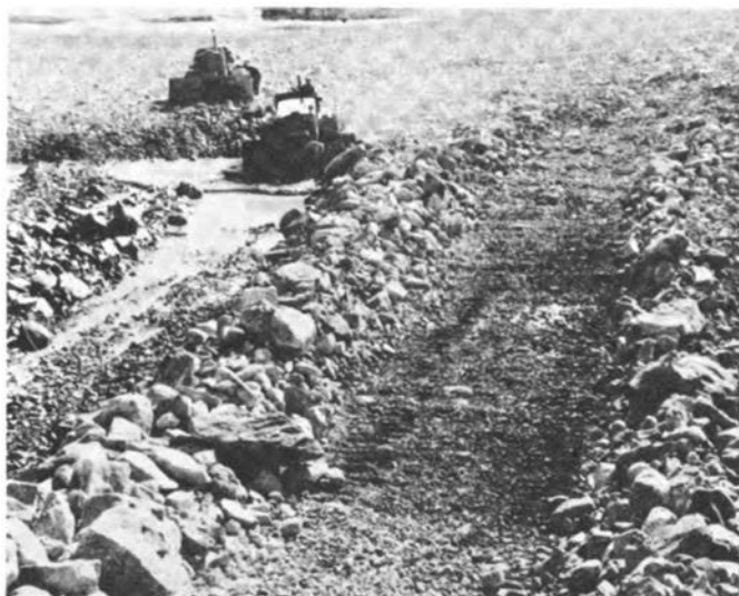
Fig. 2. Bulldozers stockpiling coarse fill from the active zone
