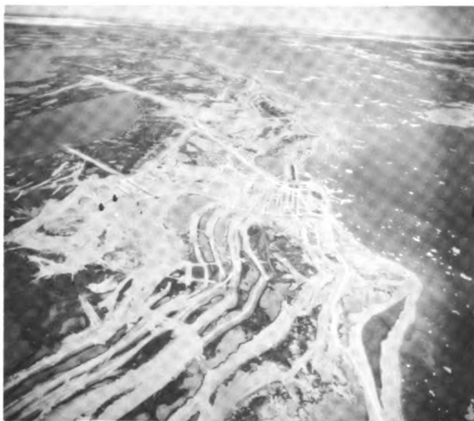
Fig. 5. Station site in Foxe Basin. Note alignment of the longitudinal axis of buildings to the prevailing wind so as to prevent drifting between buildings
