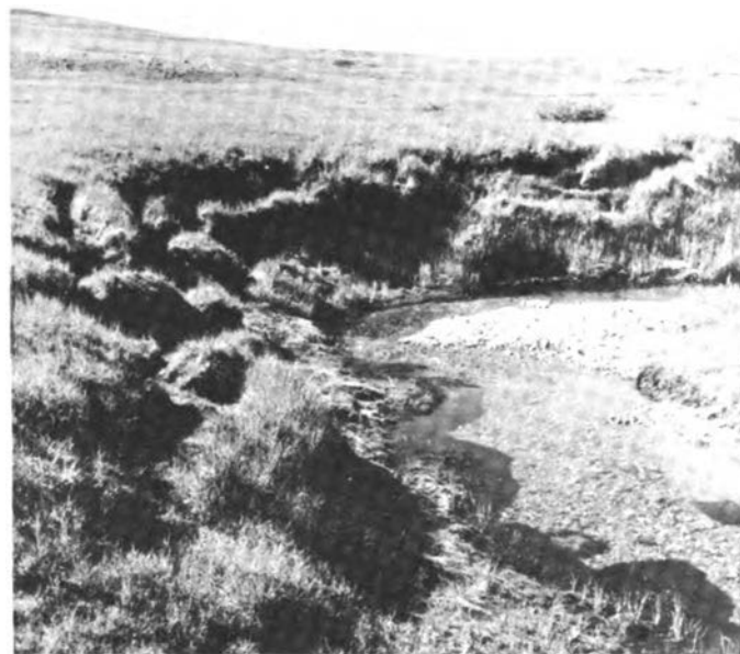
Fig. 13. Slumping and erosion of a creek bank in vicinity of Mile 22. Colluvial materials underlying the slightly sloping surface have high ice contents
