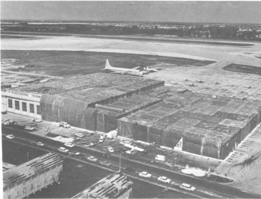
FIGURE 53 A 4-acre complex of buildings being covered with gasproof sheeting prior to fumigation. (From The Dow Chemical Company)
