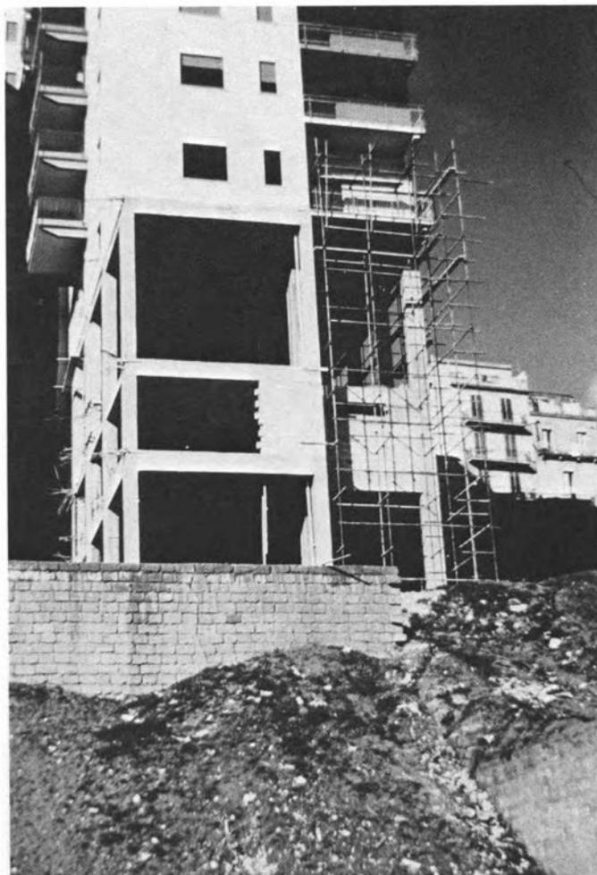
**Figure 5.** Salemi. Part of multistory, reinforced-concrete frame apartment building nearing completion. There were no outward signs of significant damage visible from the distance at which the picture was taken.
