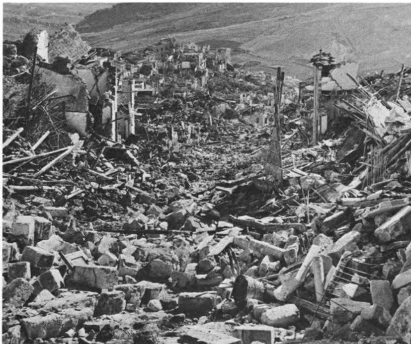
**Figure 19.** Gibellina. Complete destruction. The construction appears to have been somewhat more substantial than that in Salaparuta, but no less subject to damage. (Photograph courtesy of "Mondadori Epoca," Milan; photographers, "De Biasi - Del Grande - Lotti - Cioni.")
