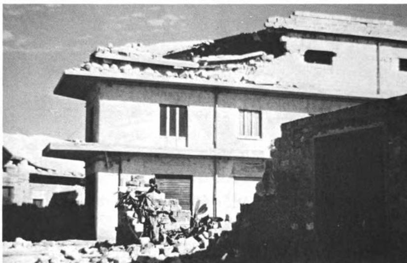
**Figure 13. Montevago. Newer construction with cut-stone masonry, concrete lintels, and reinforced-concrete floor slabs.**
