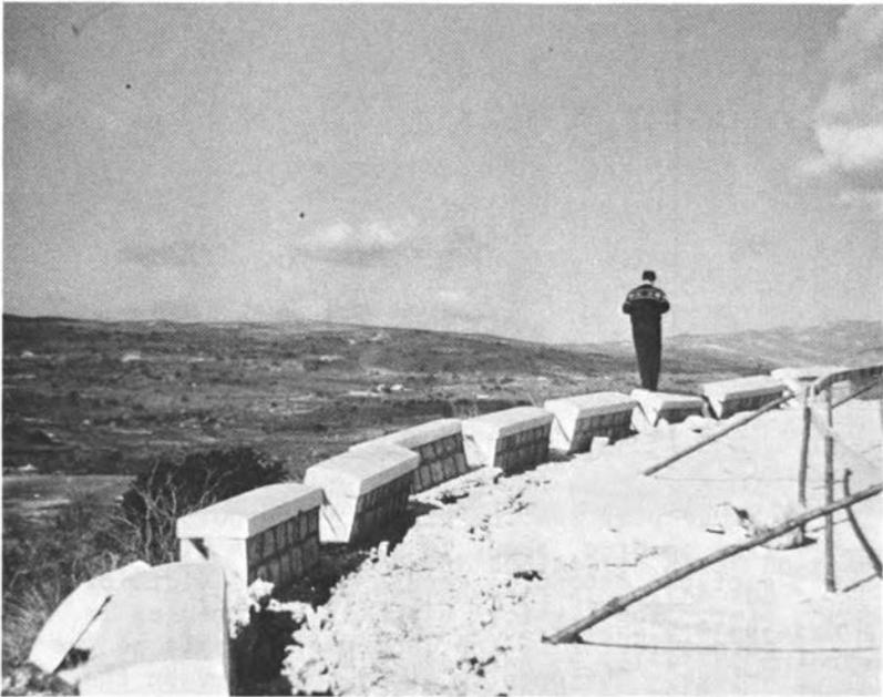
**Figure 28.** Road between Salemi and Montevago. Masonry guard walls on filled road shoulder shifted or overturned; cracks in road surface.
