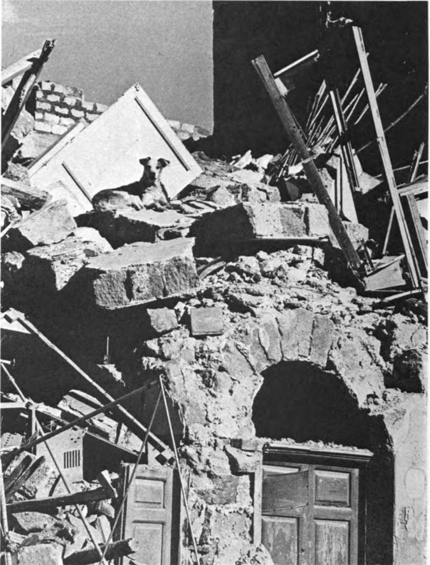
Figure 22. Collapsed building, showing the very heavy but weak masonry, heavily plastered and filled above the arch construction, the stones joined by very poor mortar. (Photograph courtesy of "Mondadori Epoca," Milan; photographers, "De Biasi - Del Grande - Lotti - Cioni.")
