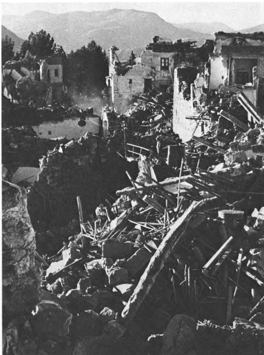
**Figure 21.** Collapsed houses, showing detail of some of the old forms of coarse masonry construction and building materials. (Photograph courtesy of "Mondadori Epoca," Milan; photographers, "De Biasi - Del Grande - Lotti - Cioni.")
