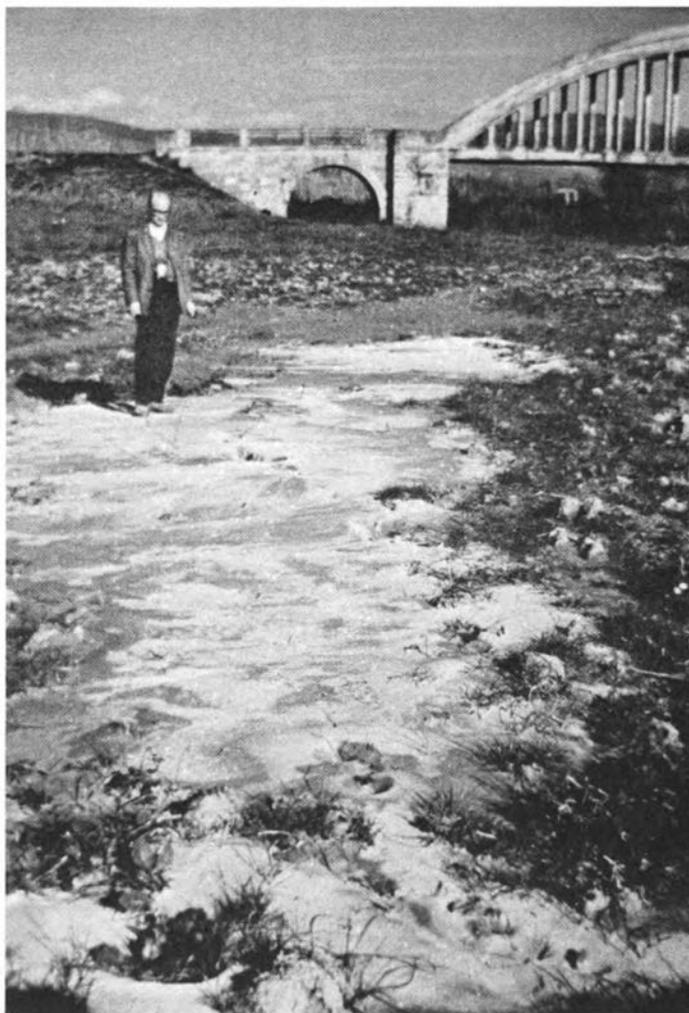
**Figure 30.** Sandboil area on the north bank of the Belice River, west of the bridge shown in Figure 26. The line of the sandboils is approximately east-west.
