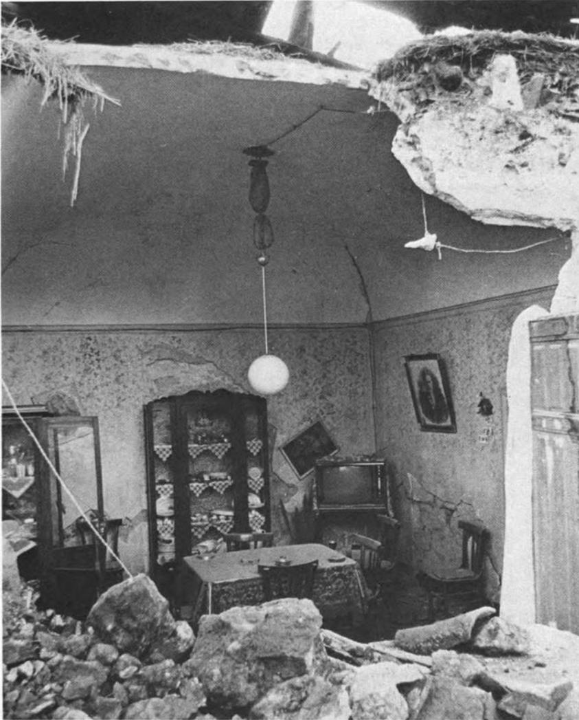
Figure 23. A dining room. Some pictures on the wall and dishes in the cabinets were displaced, but the television set, the cabinets themselves, and other furnishings do not appear to have been harmed. The exterior heavy masonry wall, however, and evidently part of the roof have completely collapsed. (Photograph courtesy of "Mondadori Epoca," Milan; photographers, "De Biasi - Del Grande - Lotti - Cioni.")
