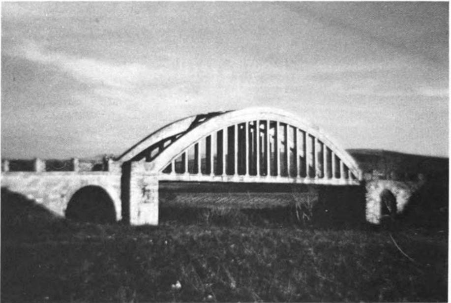
**Figure 26.** Highway bridge over the Belice River on road between Santa Margherita di Belice and Salaparuta. Reinforced-concrete tied-arch and suspenders; resting on cut-stone masonry abutment piers; span about 40 meters. The bridge suffered no apparent serious damage, and was in regular use by moderately heavy truck traffic. (View of west side of bridge).
