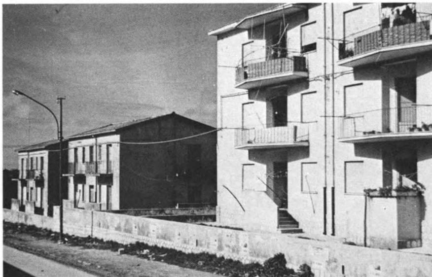
**Figure 14.** Outskirts of Montevago. Masonry and reinforced-concrete slab construction. No apparent great damage.
