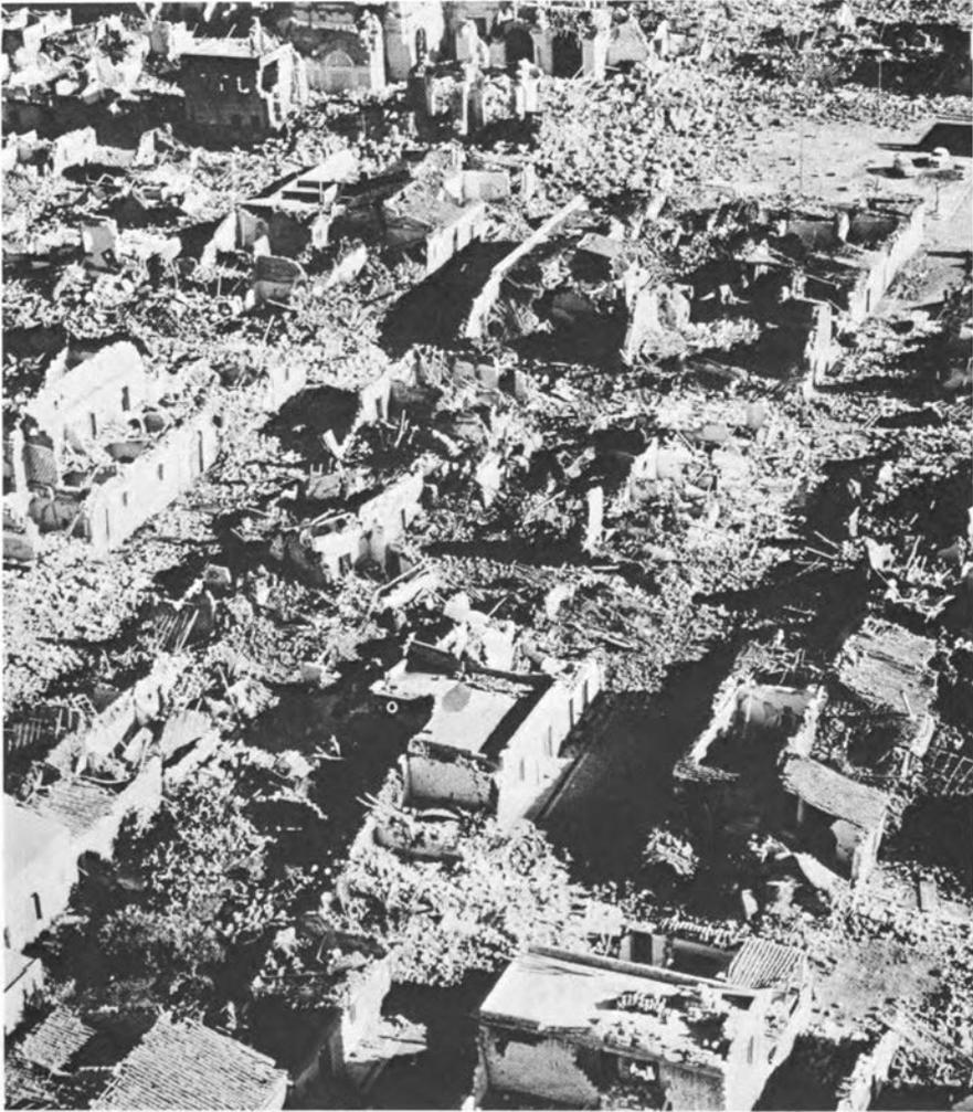
Figure 11. Montevago. At least two forms of construction are visible: an old rough masonry with pole-supported tile roofs, and a newer cut-stone masonry with reinforced-concrete floors and roofs. The newer form seems to have fared somewhat better; nevertheless, the destruction in this view is almost complete. (Photograph courtesy of "Mondadori Epoca," Milan; photographers, "De Biasi - Del Grande - Lotti - Cioni.")
