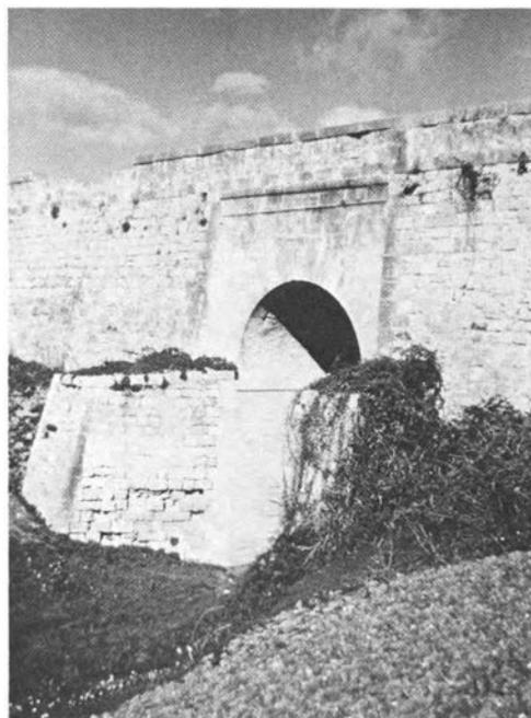
Figure 24. Near Salemi. Old highway bridge. No outward signs of great damage, but we were told that the bridge was to be removed and replaced by a culvert and fill.
