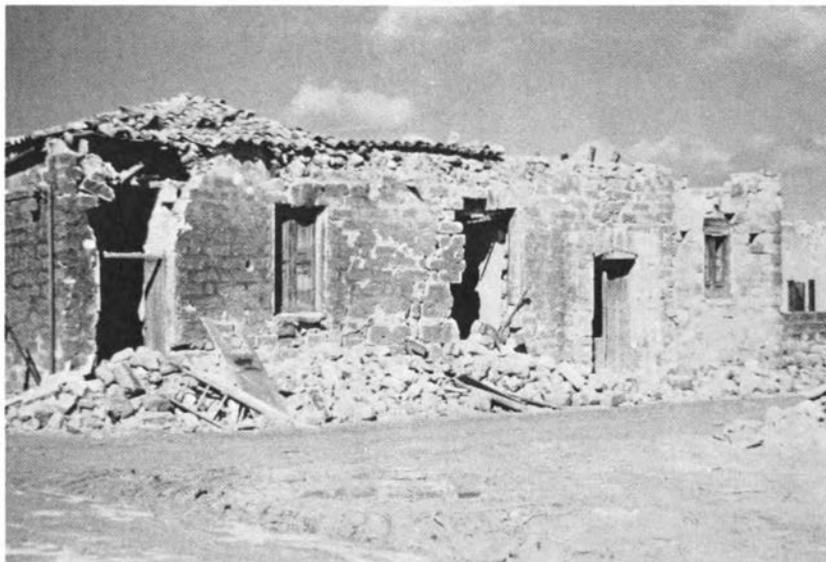
**Figure 12. Montevago. Older type of construction; rough masonry with pole-supported tile roofs.**
