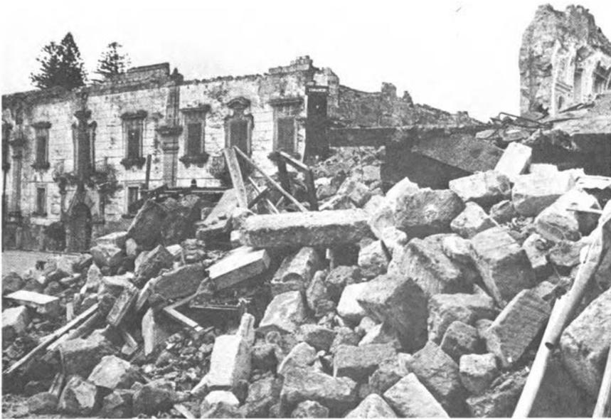
Figure 7. Santa Margherita di Belice. After the earthquake; the "Leopard's Palace" and adjoining church (compare Figure 6). The clock and parapet wall on the palace have fallen, but the facade still stands. The church is in complete ruins. (Source: "Scafidi" photographic agency, Palermo.)
