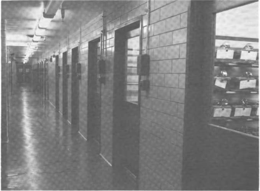
FIGURE 3 Clean corridor. The exit from the clean receiving area is on the left. The doors at the ends of the corridor are for emergency use only and are sealed with tape. The boxes to the right of each are clock-controlled switches for the lights in the room. The protrusion on the conduit leading from these boxes is a conduit that allows the insertion of an expanding mastic to seal the lumen of the conduit.
