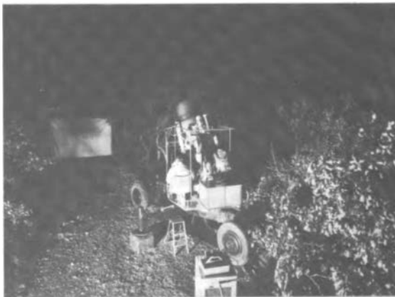
FIGURE 2 The tracking turret.
