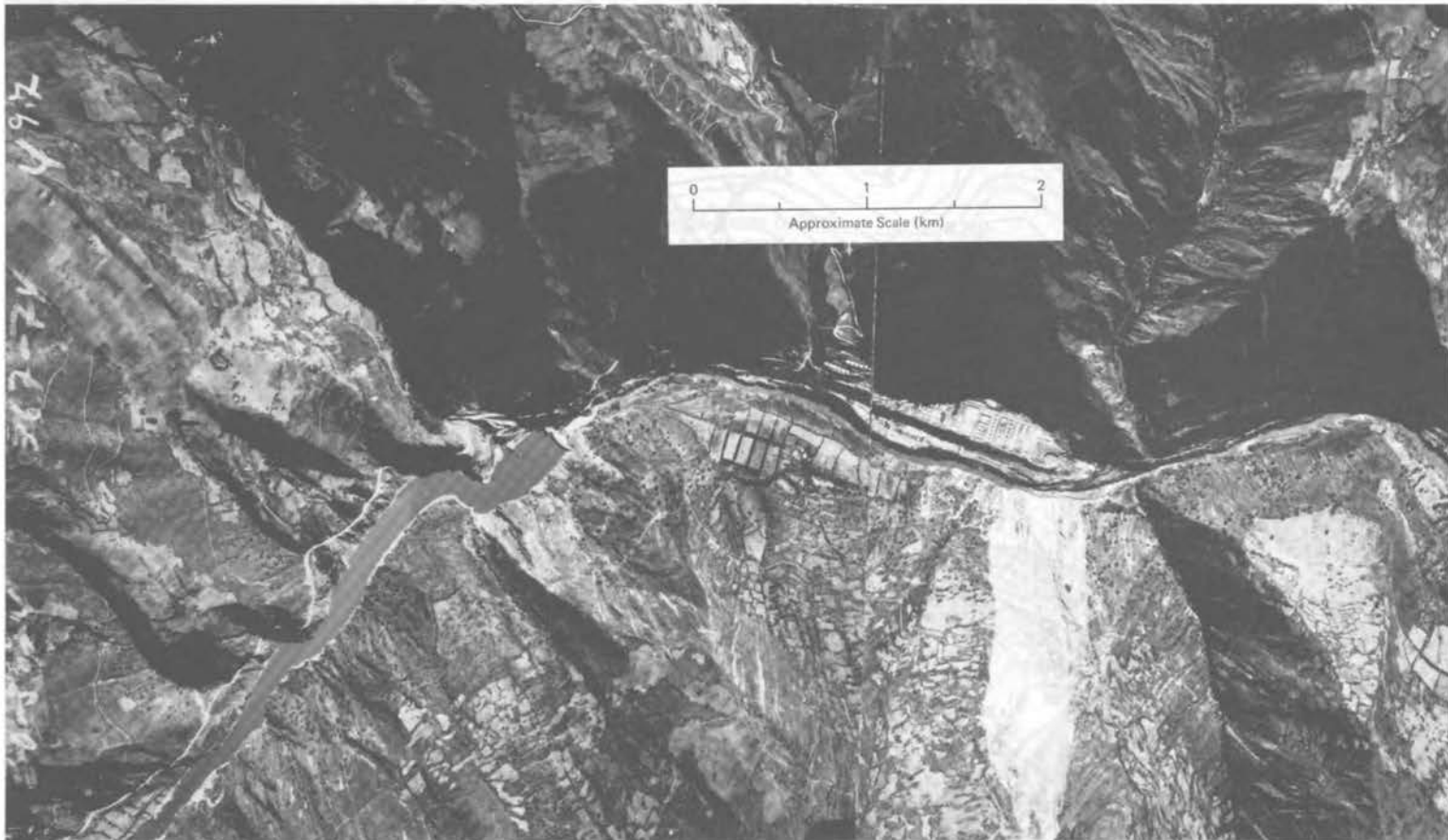
FIGURE 2. Aerial view of Tablachaca dam and electrical station, with the scarp of a 1930 landslide in the foreground. (Defensa Civil Photograph)
