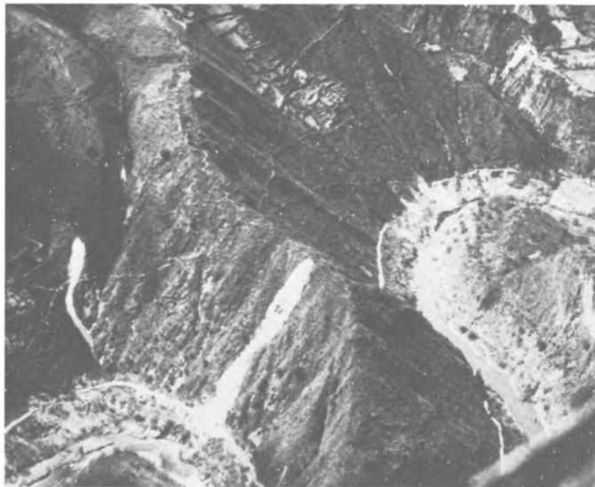
FIGURE 28. Landslide along lake shore caused by rising water.
