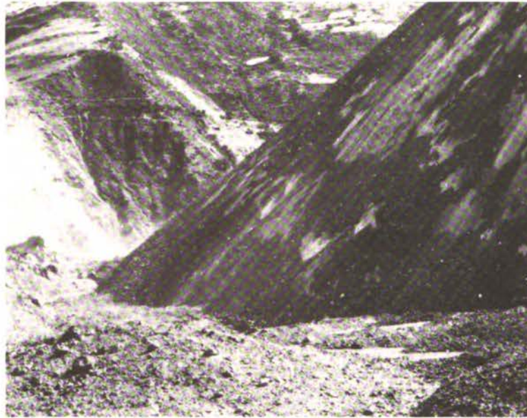
FIGURE 12. Steep slope of the Mantaro river valley opposite the main slide showing where the slide debris had run up and then fallen back down the slope. (Kojan-Hutchinson, Ref. 11)
