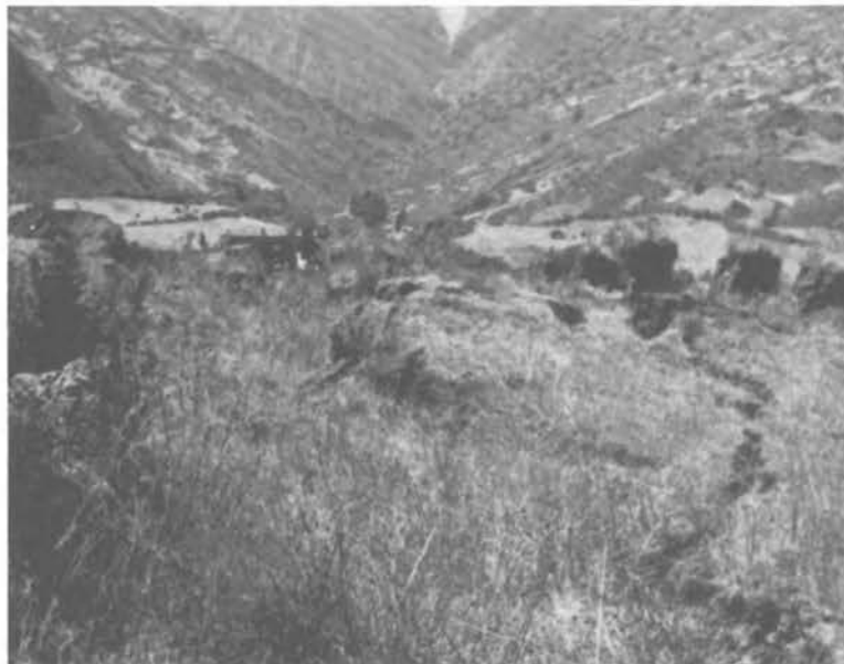
FIGURE 6. Panoramic view looking from South to North showing a system of recent fractures located 300 meters from the community center of Mayunmarca. (Photograph courtesy of Galdos Bustamante)
