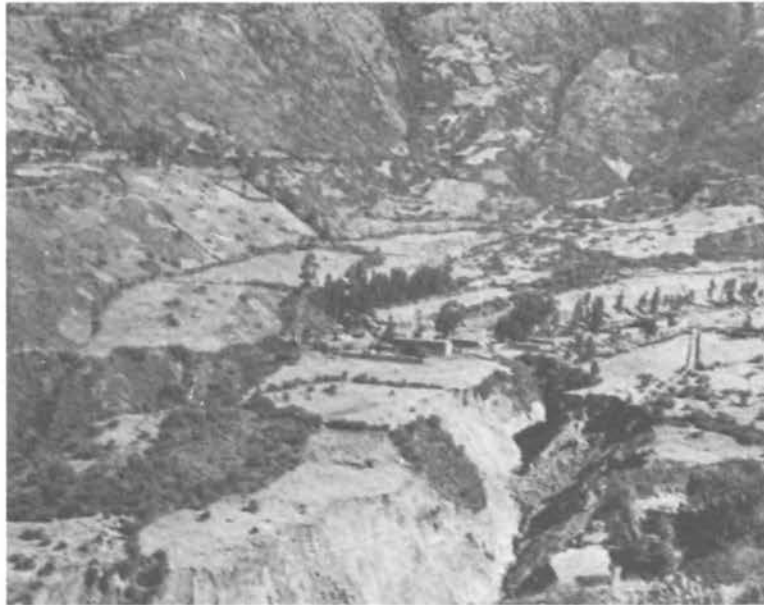
FIGURE 5. Panoramic view looking from North to South showing the community center of Mayunmarca, and the unstable slopes of the Sojosbamba ravine. (Photograph courtesy of Galdos Bustamante)
