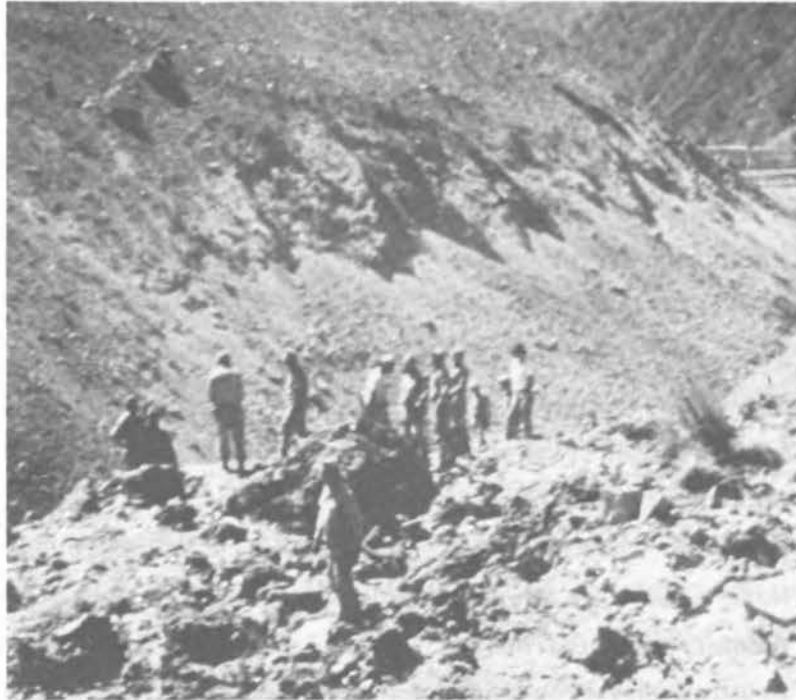
(a) Men working on slide debris before overtopping.
