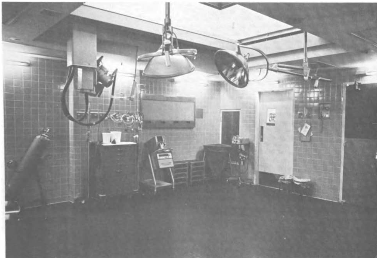
Fig. 5-A. Orthopaedic Operating Room 4 with the conventional lights off and the ultraviolet lights on. Note the UV light mounted above eye level with a protective shield. There are three lights on each wall of the room and eight lights in the overhead well. Intensity of the UV light is inversely proportional to the square of the distance. Thus, the lights at the top of the well provide adequate intensity for bactericidal effect at the level of the open surface of the operating table. The operating room adjustable, movable lights must be placed in such a way that they do not obstruct the UV light rays from the overhead well. In spite of these obstacles, however, the intensity in the room is adequate.
