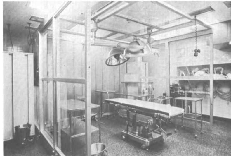
Fig. 3. Martin-Marietta Class 100 horizontal flow operating clean room.
