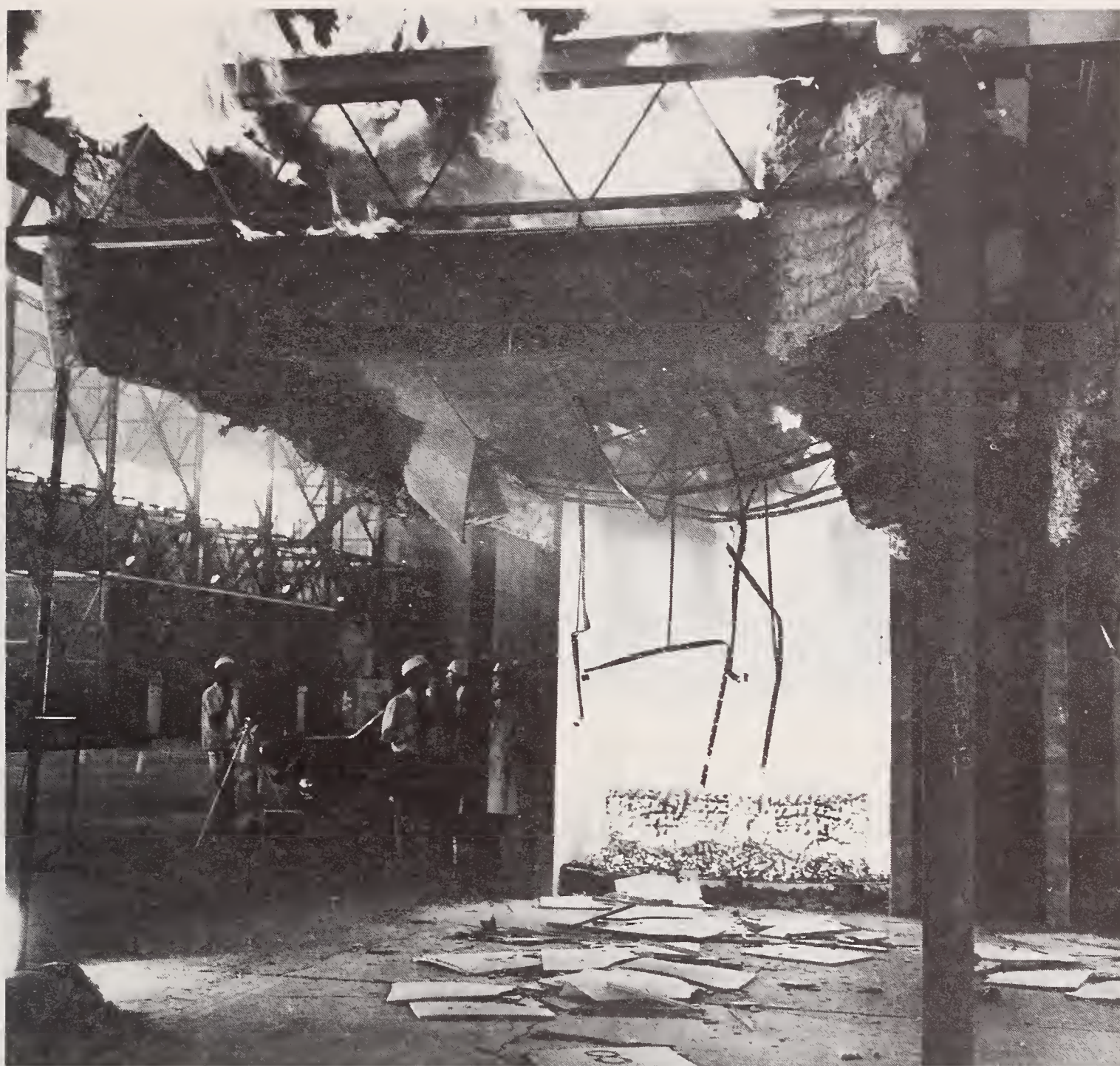
FIGURE 14 Roof construction test.
